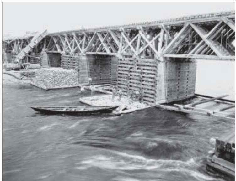
Workers built the generating station with the Winnipeg River's turbulent waters rushing close by.
