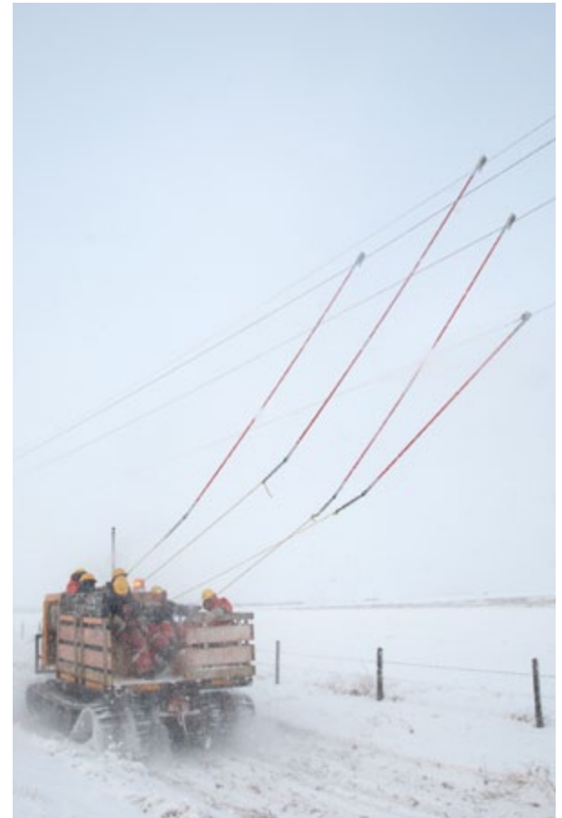
Above: Extreme and fluctuating weather conditions such as ice storms can cause ice to form on power lines. Crews use a technique called "ice-rolling" to remove the ice from power lines as quickly as possible to prevent equipment breakage and loss of power. Rollers attached to the end of long poles are pulled along the power lines cracking the ice off as they go.
