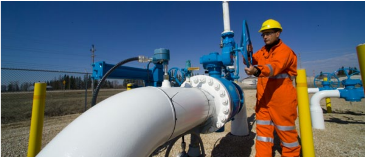
Left: Field worker from Gas Apparatus Maintenance and Control operates a valve at the gate station which supplies natural gas to the Selkirk Generating Station.
