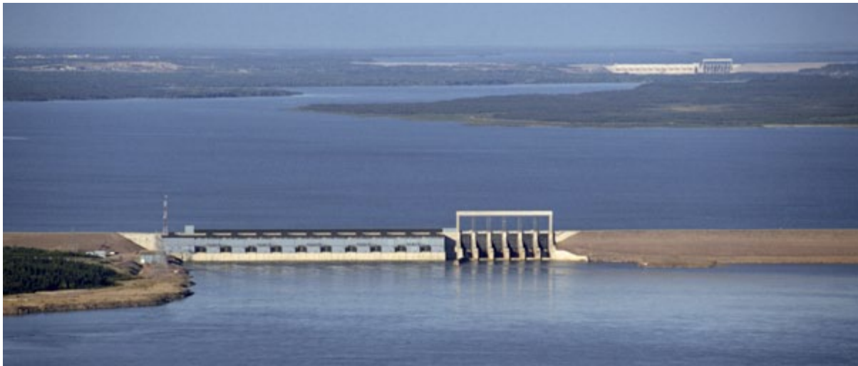
Left: The Nelson River featuring Long Spruce Generating Station with Kettle Generating Station in the background.
