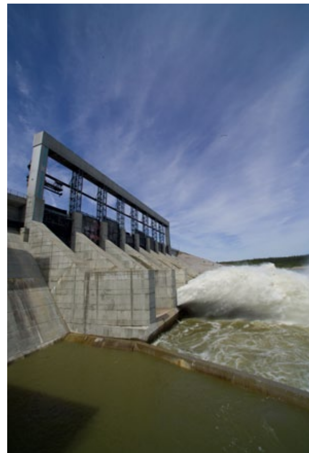
Above: The spillway at Kettle Generating Station located on the Nelson River.
