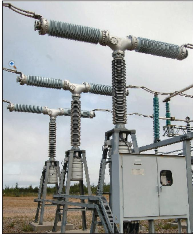
For circuit breakers, the operating mechanism, contact performance, arc extinction and service record sub-condition parameter inputs were supplied by data and/or corrective maintenance records obtained from an electronic maintenance database(s) whereas much of the insulation sub-condition parameter inputs were supplied by actual test data. Additional factors such as obsolescence, known design flaws or performance issues were also accounted for in the AHI.
