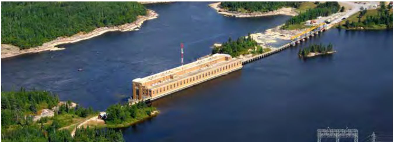
Slave Falls Generating Station is located on the Winnipeg River about 35 kilometres east of Lac du Bonnet.
