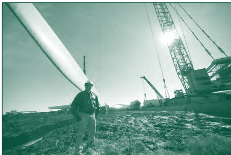
Using the world's tallest crane, the first wind turbine's 80 metre high steel tower was raised, followed by the blades, which are longer than a 747 jet airplane.
