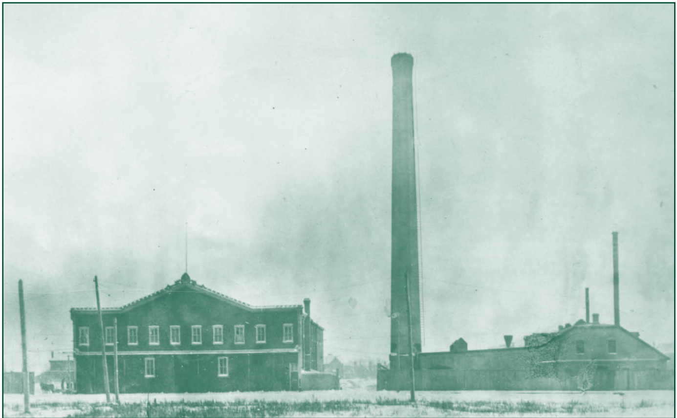
The Assiniboine steam plant's capacity was originally measured in horsepower, a unit of power in the Imperial system equal to 550 foot-pounds per second, which is approximately 746 watts (W). A watt is a unit of power in the metric system. The Assiniboine steam plant's capacity in 1895 was rated at 750 horsepower. The term horsepower was initially used to describe the power of pumps, beginning in about 1806. As time passed, horsepower was used to describe the power of a variety of mechanical devices, such as steam engines.
