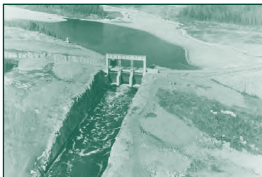
The Missi Falls Control Dam at the natural outlet of Southern Indian Lake controls the water outflow from the lake. The lake's level was raised three metres as part of the Churchill River Diversion Project.
