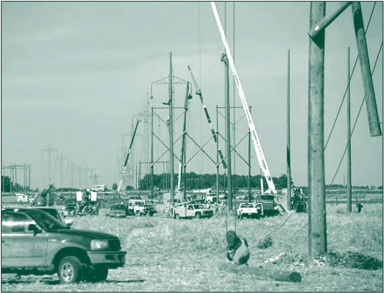
Some of the 19 steel towers that collapsed when tornado-like winds hit the Grosse Isle area were replaced temporarily by wood poles in order to get the electricity flowing again. In about seven weeks, all steel towers were replaced and the Bipoles 1 and 2 transmission line systems were back to normal.
