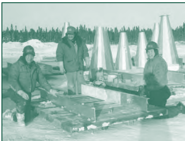
Workers of Split Lake-Comstock Joint Venture (photo above) assemble foundations for one of the tubular steel towers used on the new 138-kV transmission line from Kelsey Generating Station to Split Lake (photo right). It was cold for the workers, but work could be carried out and equipment could be moved in and out of the area more easily in winter because the ground was frozen.
