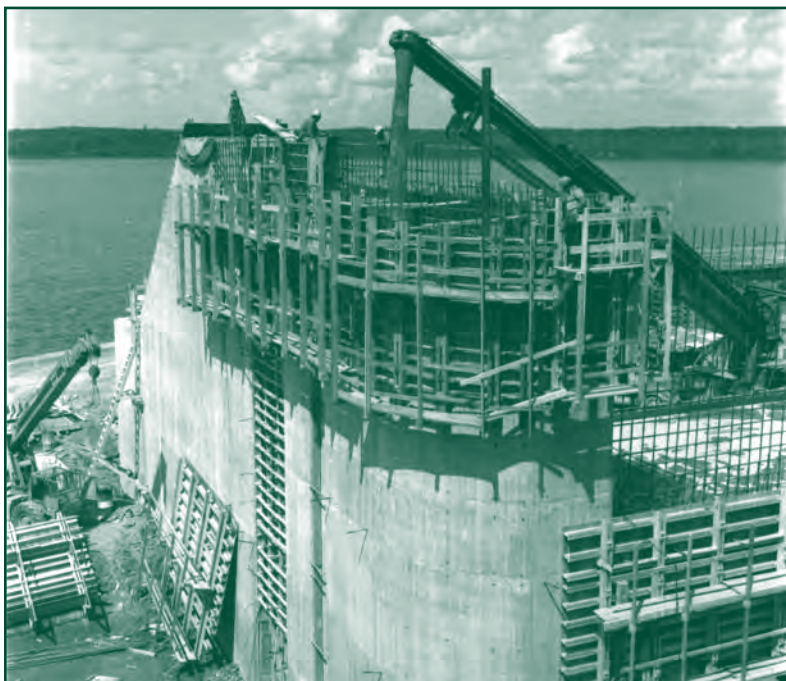
Because of concrete deterioration after more than half a century of continuous use, major rehabilitation work at Great Falls Generating Station began in 1978. The work included replacement of the spillway and west non-overflow dam, as well as concrete repairs to the powerhouse.
