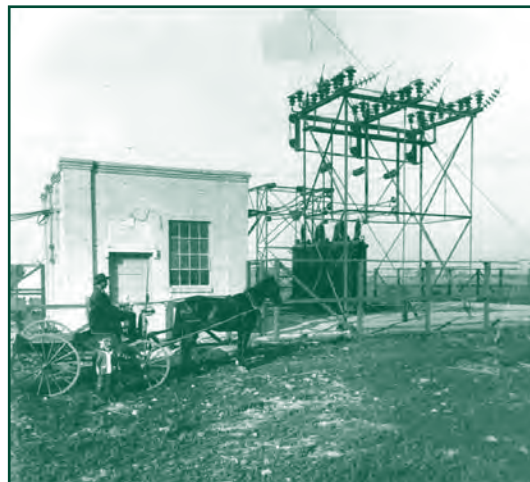
The Portage la Prairie substation in 1920 was known as MPC Substation No. 2. This structure terminated MPC's first transmission line which linked Winnipeg to Portage la Prairie. The substation was energized on August 21, 1920. Power was supplied by Pointe du Bois Generating Station.
