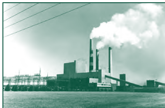
Brandon Generating Station was MHEB's first thermal (coal burning) generating station. With a capacity of 237 MW, it was designed to supplement the hydroelectric generating stations during periods of extreme drought.
