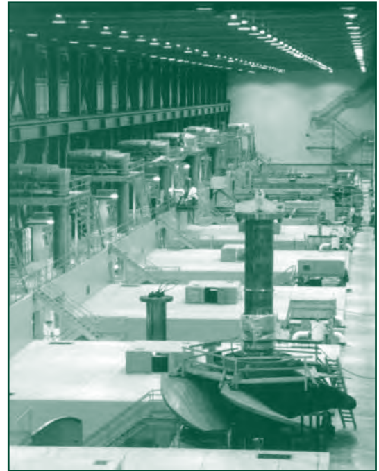
One of the turbine assemblies stood ready for installation in the Limestone Generating Station powerhouse. Each one of the 10 turbine generators at Limestone can produce 133 MW of electricity.
