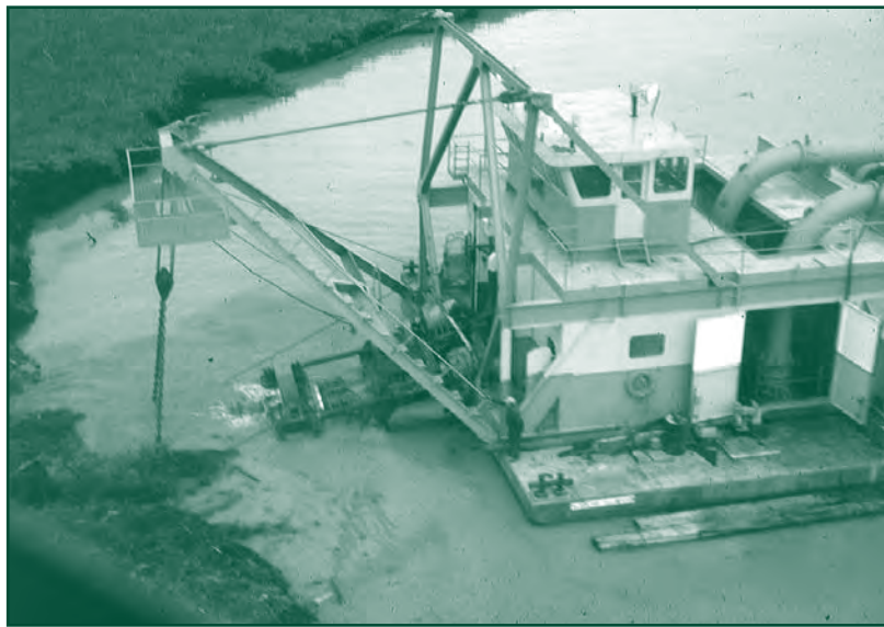
Dredging work was done on the eight-mile Channel between Playgreen Lake and Kiskittogisu Lake. The three channels were constructed as part of the Lake Winnipeg Regulation — two-mile Channel, eight-mile Channel, and Ominawin Channel — and helped to increase water flows for hydroelectric development on the Nelson River.
