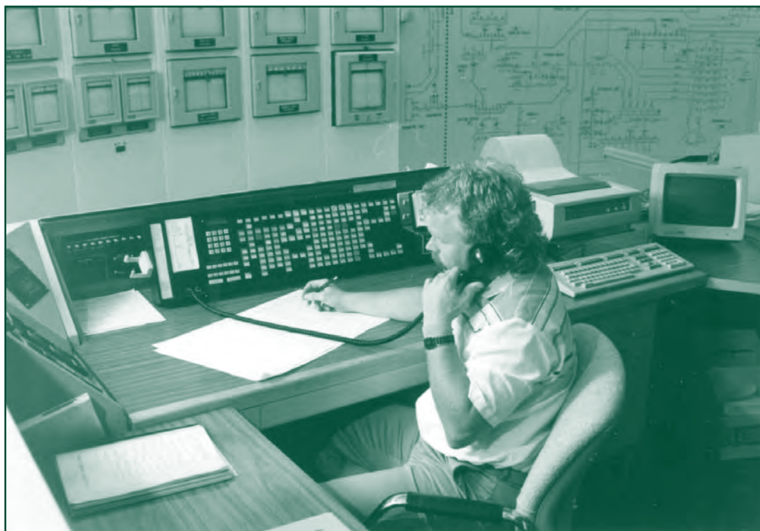
Twenty-four hours per day, seven days a week, Manitoba Hydro's System Control Centre in Winnipeg is staffed. The control centre ensures the ever-changing electricity demands of customers in Manitoba are met. Computer controls help improve system reliability and operating efficiency. The generating stations, transmission lines, and electricity exports to other utilities are monitored constantly.
