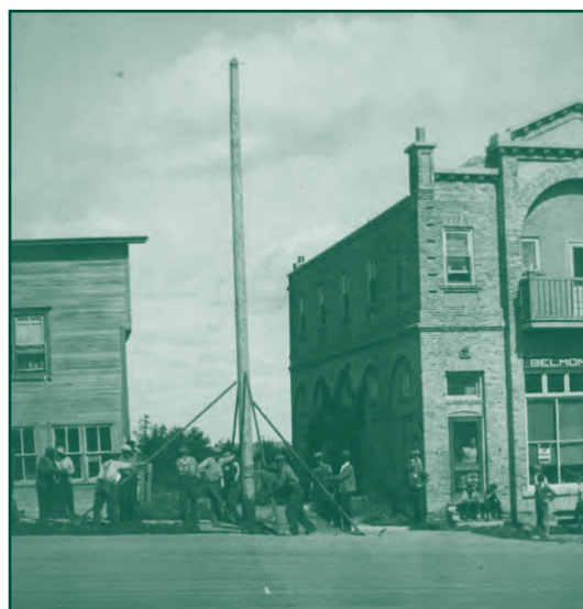
In 1936, the first pole was erected for distributing electricity in the town of Belmont, located in south-western Manitoba. The transmission line network, established for bringing electricity to various towns in Manitoba, later formed the infrastructure for the massive Farm Electrification program.
