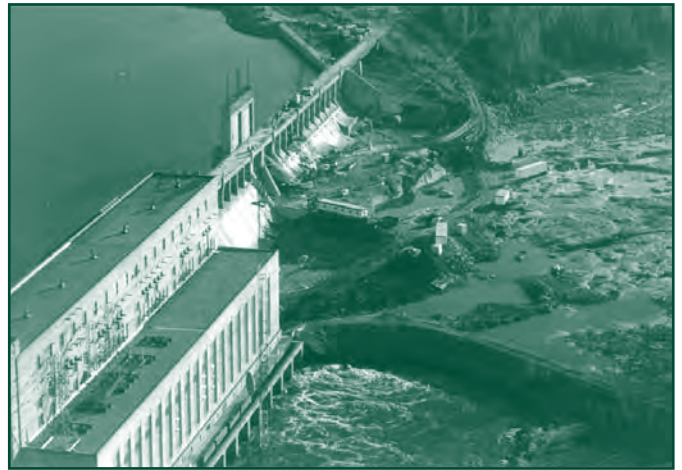
Rehabilitation work at Seven Sisters Generating Station was underway from 1979 until 1985. Major repairs were made to the spillway and sluiceway, the north dam, and the powerhouse.
