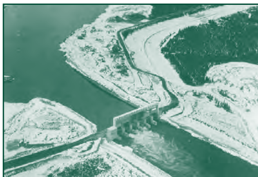
The Notigi Control Dam, also part of the Churchill River Diversion Project, is located on the Rat River and controls the flow of water from the Churchill River into the Burntwood-Nelson river system.
