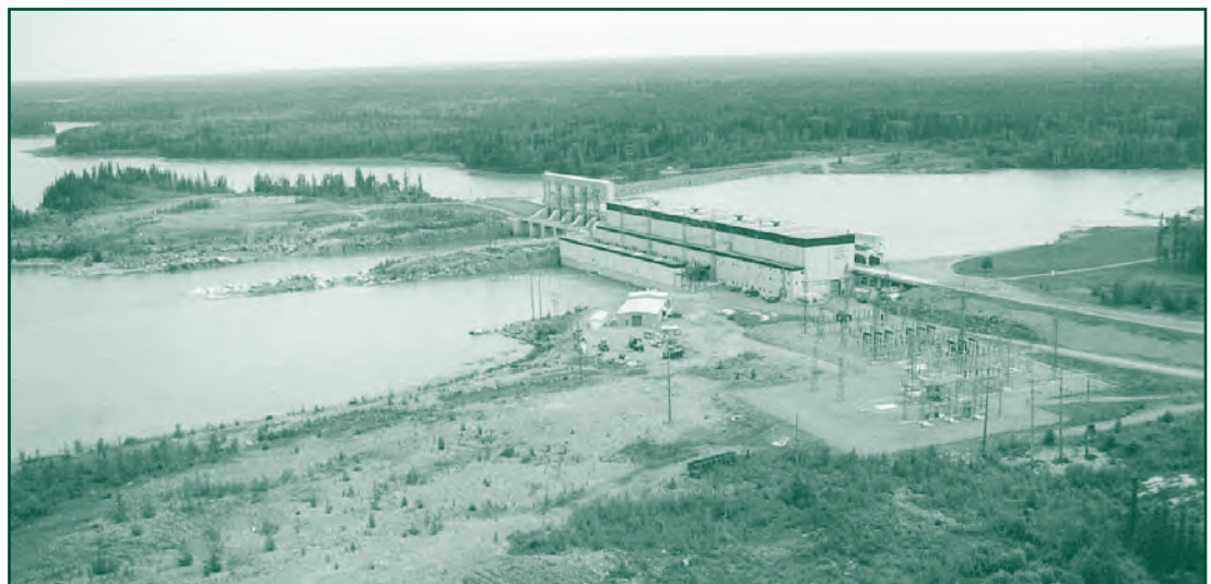
Jenpeg Generating Station and Control Dam on the Nelson River. Although Jenpeg does produce electricity, its primary purpose is to control water levels in accordance with the terms of Manitoba Hydro's licence for regulating Lake Winnipeg.
