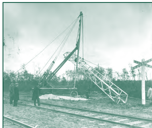
The erection of the first tower on the Manitoba Power Commission’s system took place on October 3, 1919. Witnessing the event were three of the engineers who planned MPC’s transmission line network (Winnipeg to Portage la Prairie): Mr. C. Gunn, Mr. T. Kirby and Mr. J. Rochetti, MPC’s first chief engineer.
