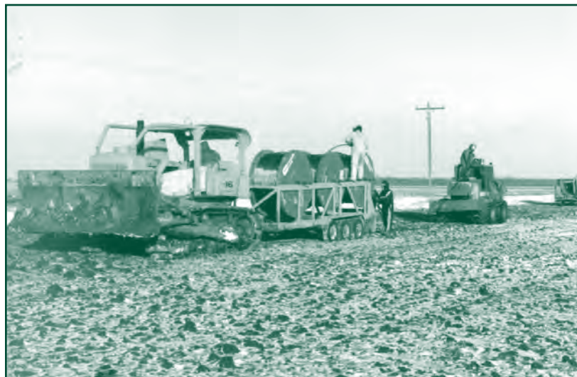
Manitoba Hydro's crews installed underground power lines between the towns of Manitou and Darlingford. This was a part of the Rural Underground Distribution program, which was established to help minimize power outages in areas of the province susceptible to ice storms.
