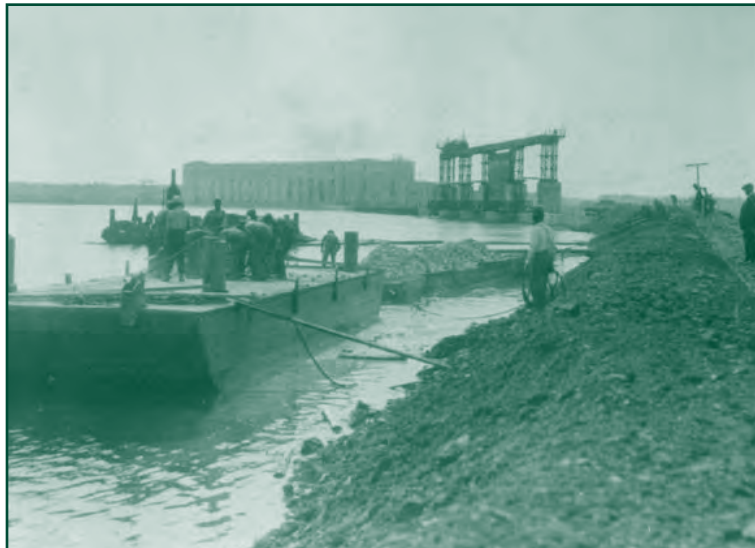
Development work at Great Falls on July 13, 1928. Work crews used barges to place material on the rockfill dam.
