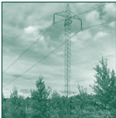
Manitoba Hydro's High Voltage Direct Current transmission lines, which follow a route almost 900 km long, are among the world's longest.
