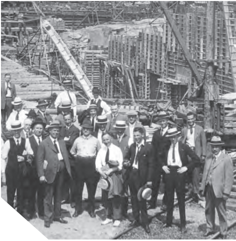
Great Falls Generating Station construction, circa 1920.
