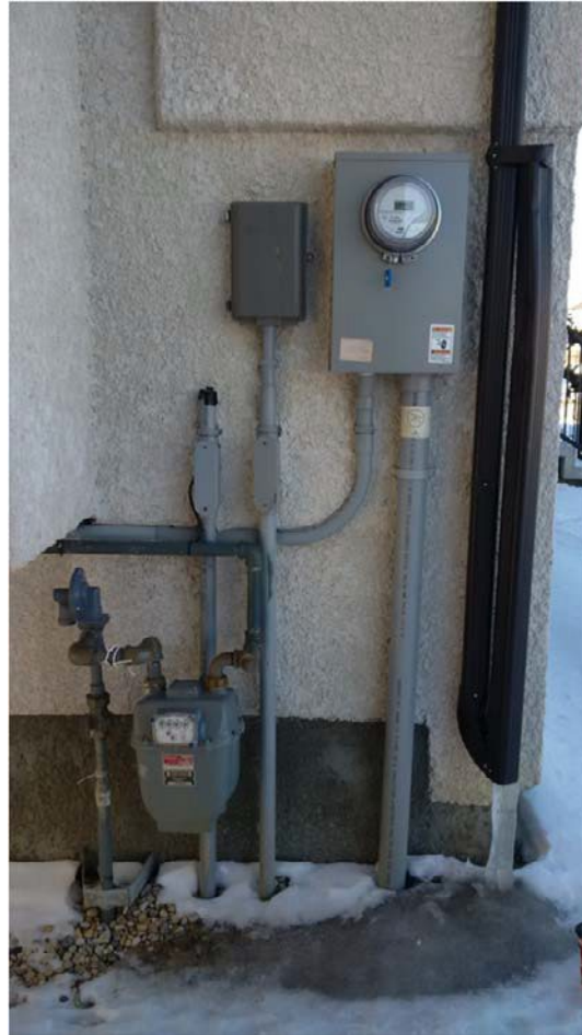
Figure 4A – Photo of Example Left Side Four-Party Utility Arrangement
