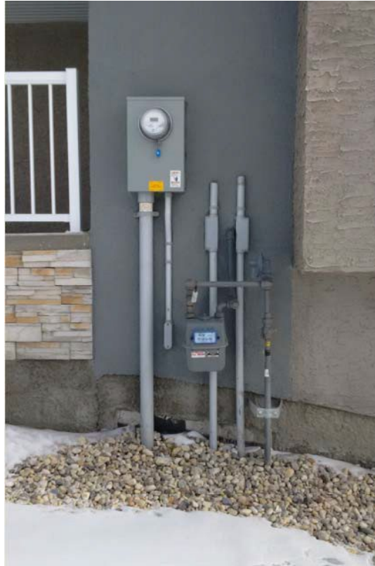
Figure 3A - Photo of Example Right Side Four-Party Utility Arrangement
