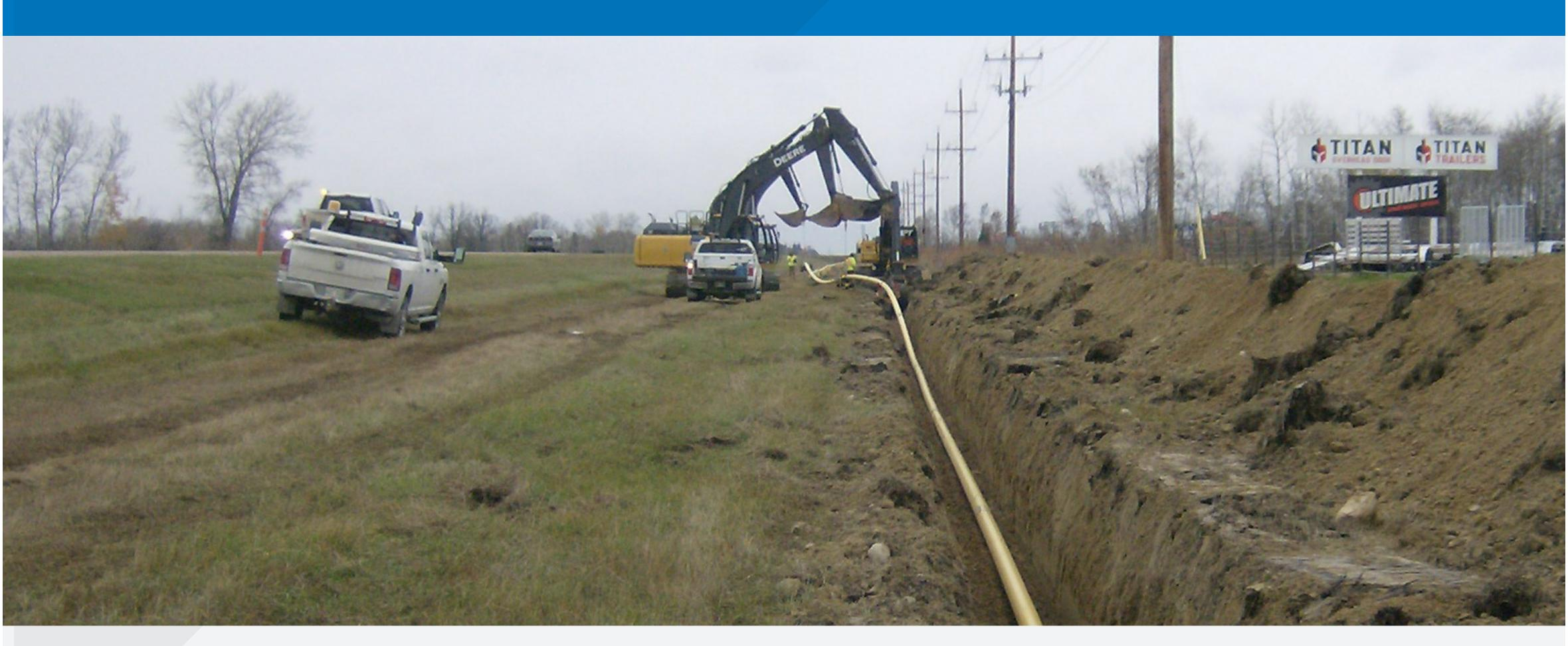
**Trenching** involves digging a long narrow hole in the ground and placing the pipeline within it.
