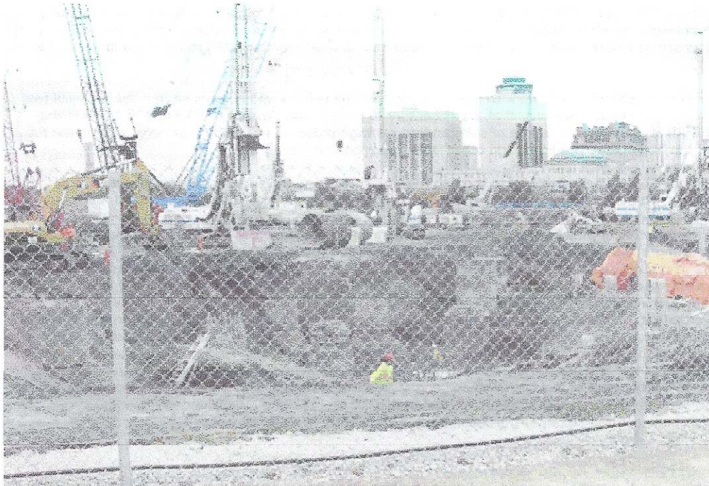
2009 excavation at the CMHR site showing one of the cavernous holes that was dug through the ancient village layers for caps for pilings. (Photograph by E. Leigh Syms) 2009 excavation at the CMHR site showing one of the cavernous holes that was dug through the ancient village layers for caps for pilings. (Photograph by E. Leigh Syms)
