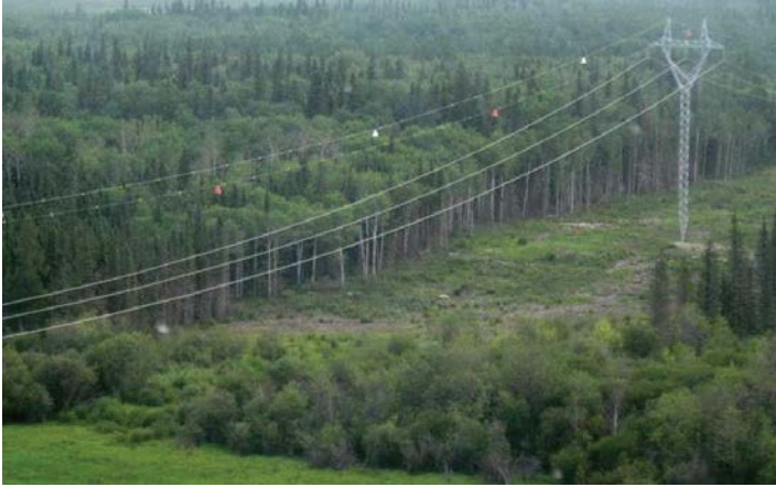
Photo 15: Bird Diverters on a Transmission Line
