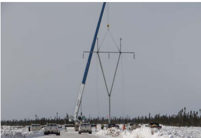
Photo 3: Installation of a Transmission Structure for the Construction Powerline
