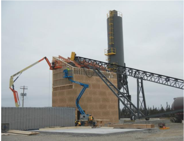
Photo 4 Installation of concrete batch plant at Keewatinohk
