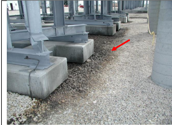
Photo 1: Grey-black PHC, PAH, and/or PCB soil staining
