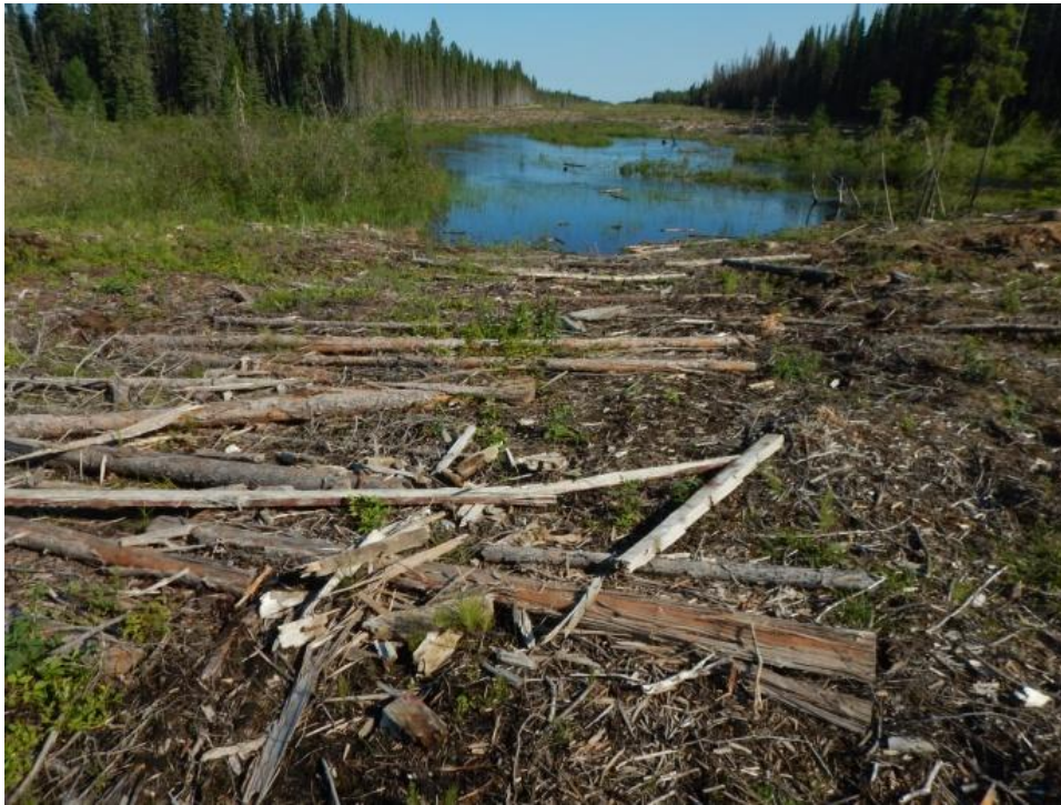
Photograph 4-5c. Logs used at water crossing to reduce surface erosion.
