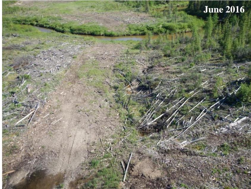
Photo 5. N1-Aqua-133 (unnamed tributary of South Moswakot River). Channel runs within the riparian buffer zone in the RoW, prone to erosion, June 2016.
