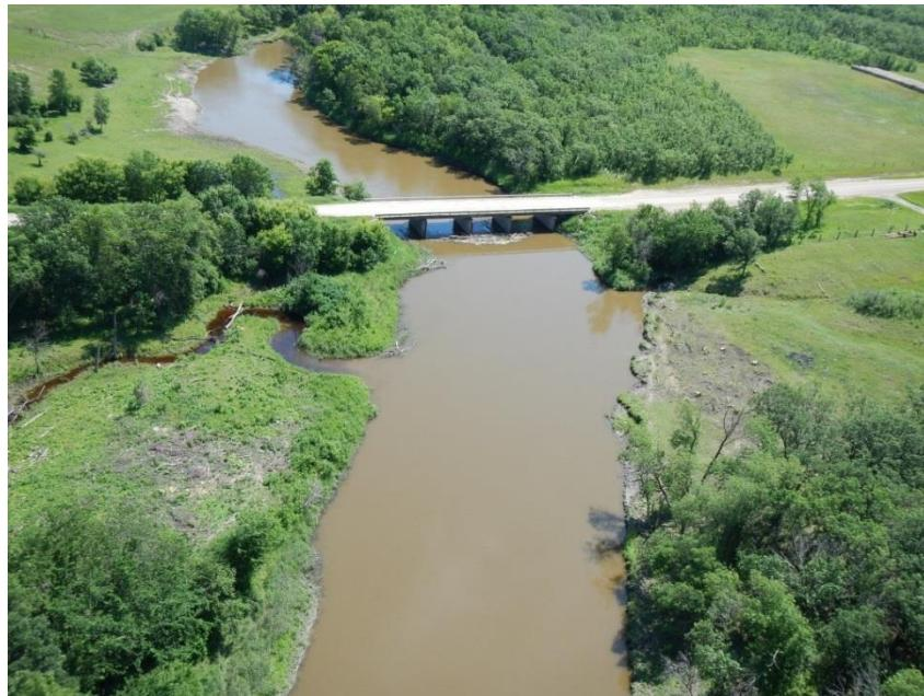
Photo 27. S1-Aqua-112 (Whitemud River). Woody debris accumulated against supports of bridge immediately downstream of the RoW, June 2016.
