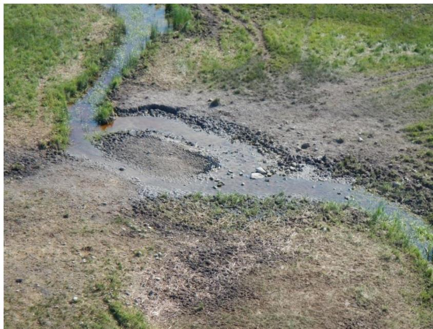
Photo 26. C1-Aqua-125 (German Creek). Erosion of the stream at the vehicle and cattle crossing, June 2016.
