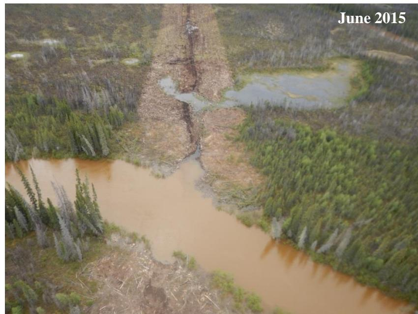
Photo 2. N1-Aqua-129 (Limestone River). Channel within RoW is subject to erosion, June 2015.
