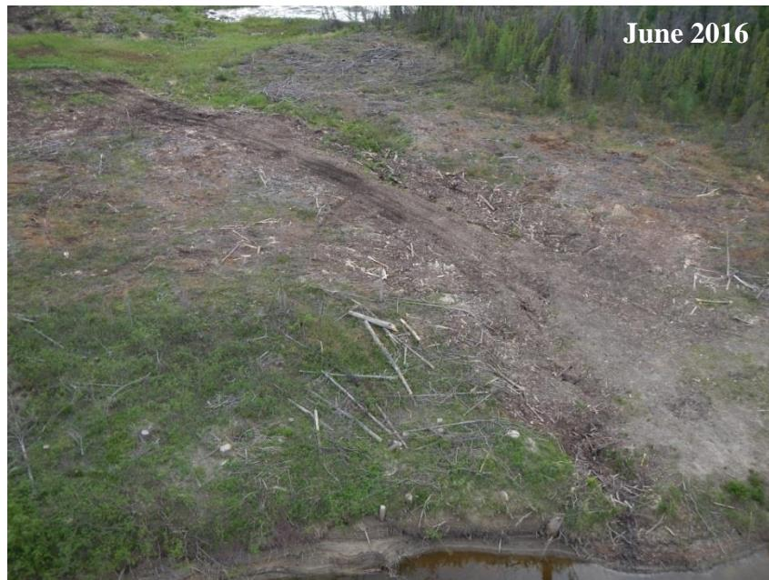
Photo 3. N1-Aqua-129 (Limestone River). Channel within RoW is subject to erosion, June 2016.
