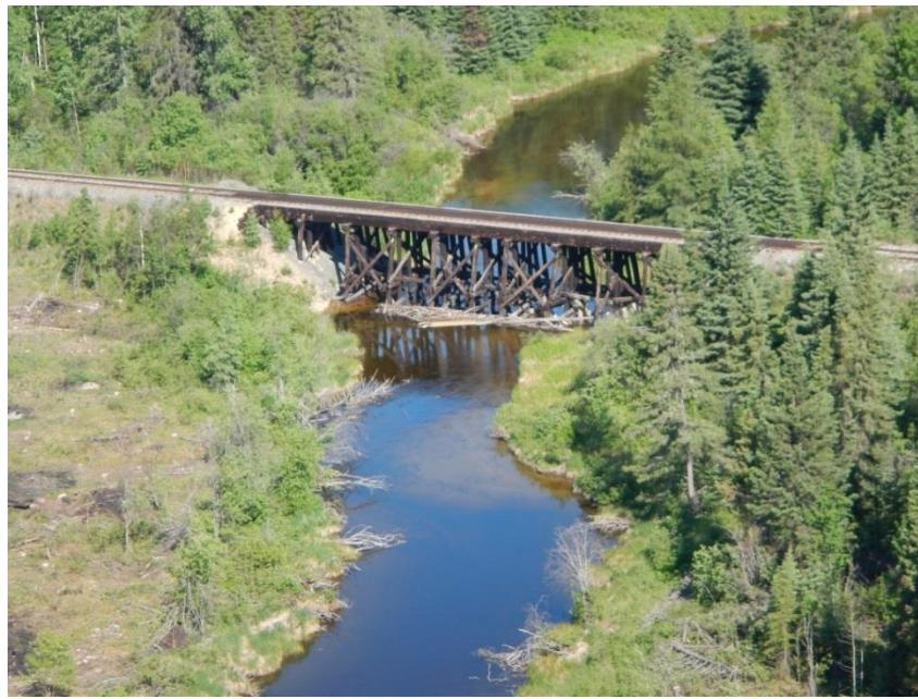
Photo 20. N2-Aqua-166 (unnamed tributary of Gormley Creek). Woody debris accumulated against supports of bridge immediately downstream of the RoW, June 2016.
