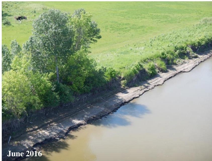
Photo 24. N3-Aqua-134 (Saskatchewan River). Shrubs and forbes becoming well established on the southern bank, June 2016. Slumping does not appear to have increased since June 2015.
