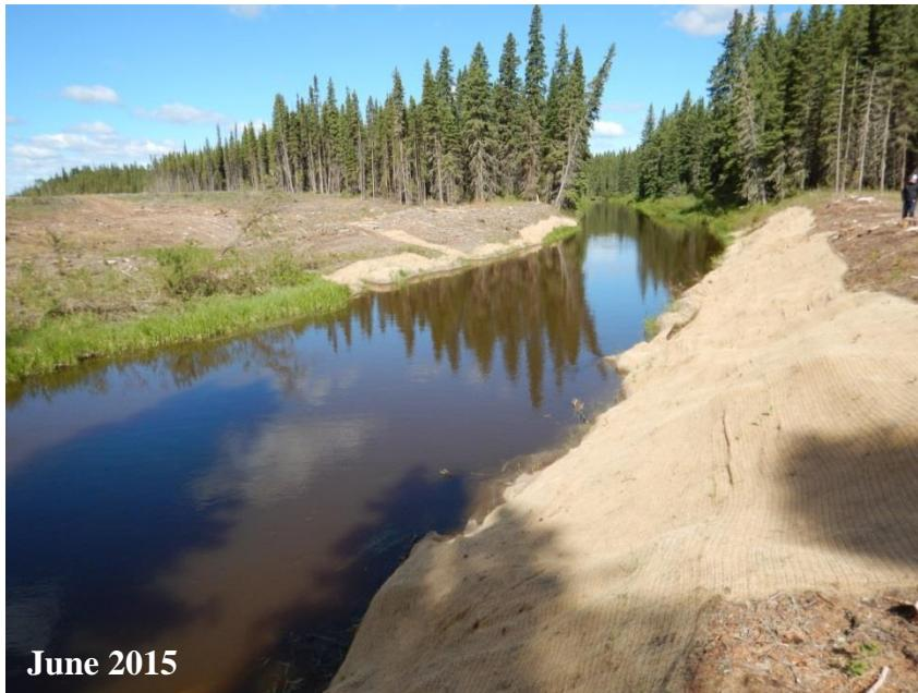
Photo 21. N3-Aqua-103 (Mitishto River). Excessive clearing in RBZ and exposed soil prone to erosion protected by erosion control matting, June 2015.
