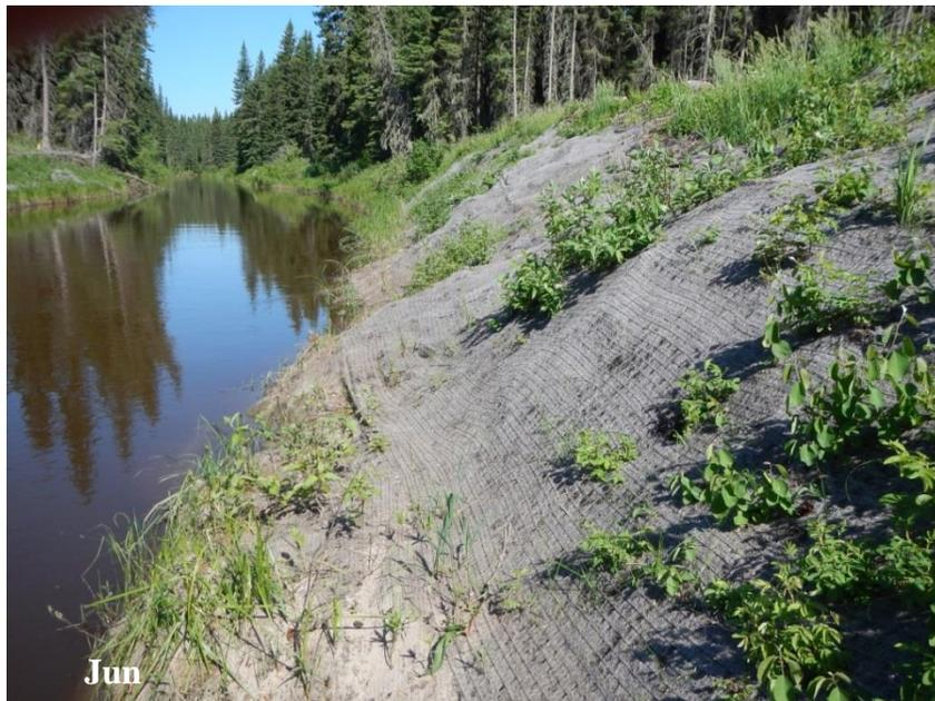
Photo 24. N3-Aqua-103 (Mitishto River). Shrubs and forbes becoming established on the steep eastern bank through erosion control matting, June 2016. No erosion was detected.
