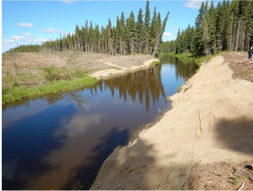
Photo 23. N3-Aqua-103 (Mitishto River). Excessive clearing in RBZ and exposed soil prone to erosion protected by erosion control matting, June 2015.
