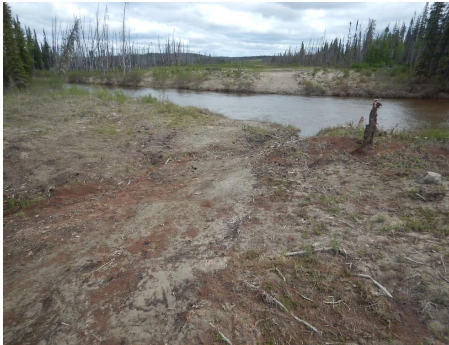
Photo 3. N1-Aqua-129 (Limestone River). Channel within RoW is subject to erosion, June 2017.
