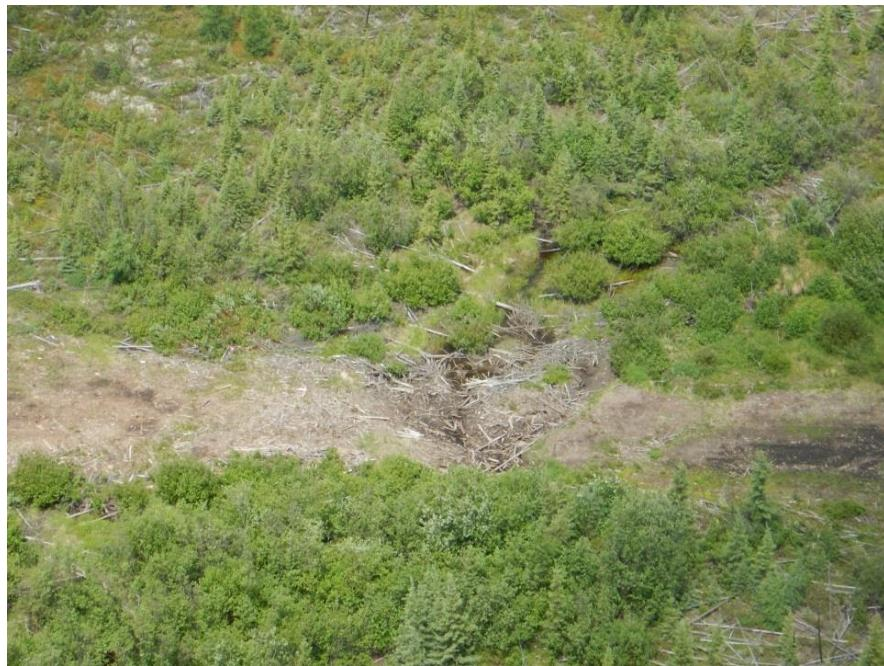
Photo 17. N1-Aqua-161 (unnamed tributary of the Burntwood River). Woody debris and slash left below the HWM and within the watercourse crossing. Marginal fish habitat but should consider removing, June 2018.
