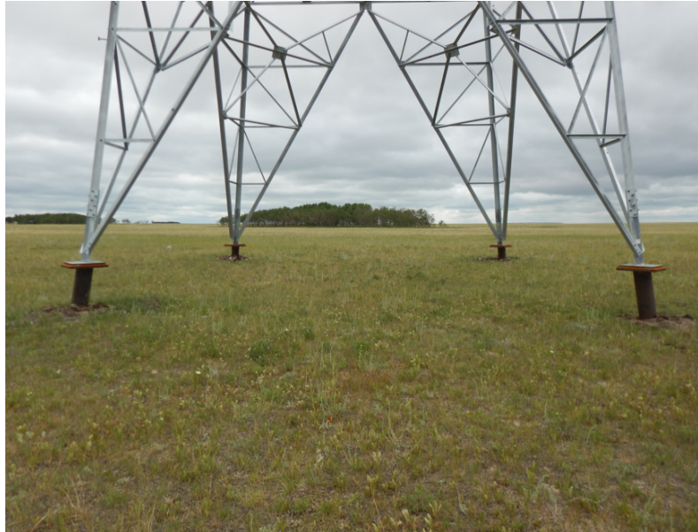
Photograph 4-6b. Tower 120 installed with minimal soil disturbance.
