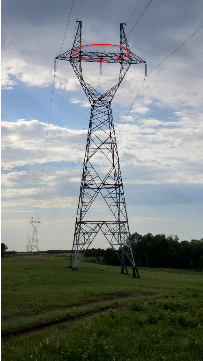
Photo 5: Perch deterrents on a transmission tower
