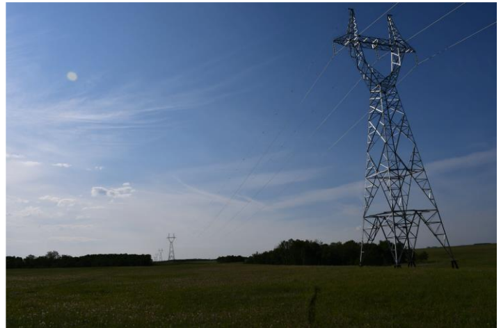
Photo 1. The Birtle Transmission Project was completed in March 2021.
