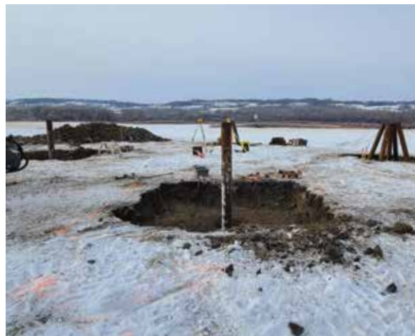
Pictured above: Earth excavated for the construction of the base of Tower 113
