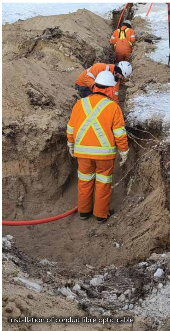
Channel digging for fibre optic cable installation
