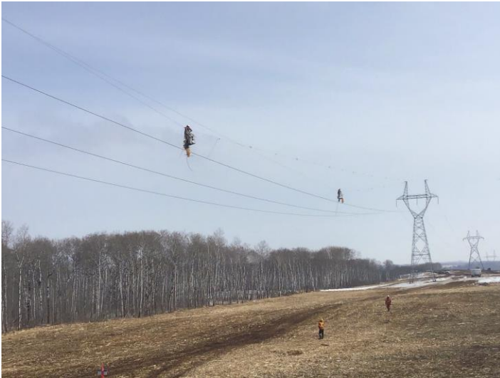
Photo 7. Grassland sites in the Spy Hill Community Pasture were outfitted with bird diverters on conductors and avian perch deterrents on the towers.
