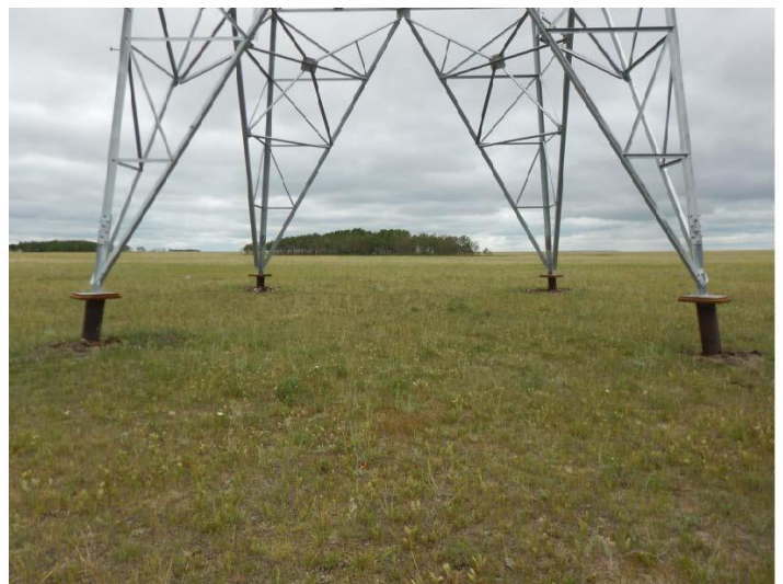
Photo 3. A tower installed in the Spy Hill Community Pasture with minimal soil disturbance.
