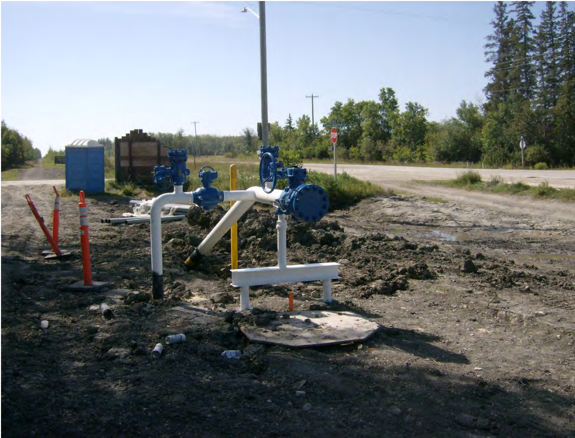
Photo 2-2: Example of control point and pig launcher
