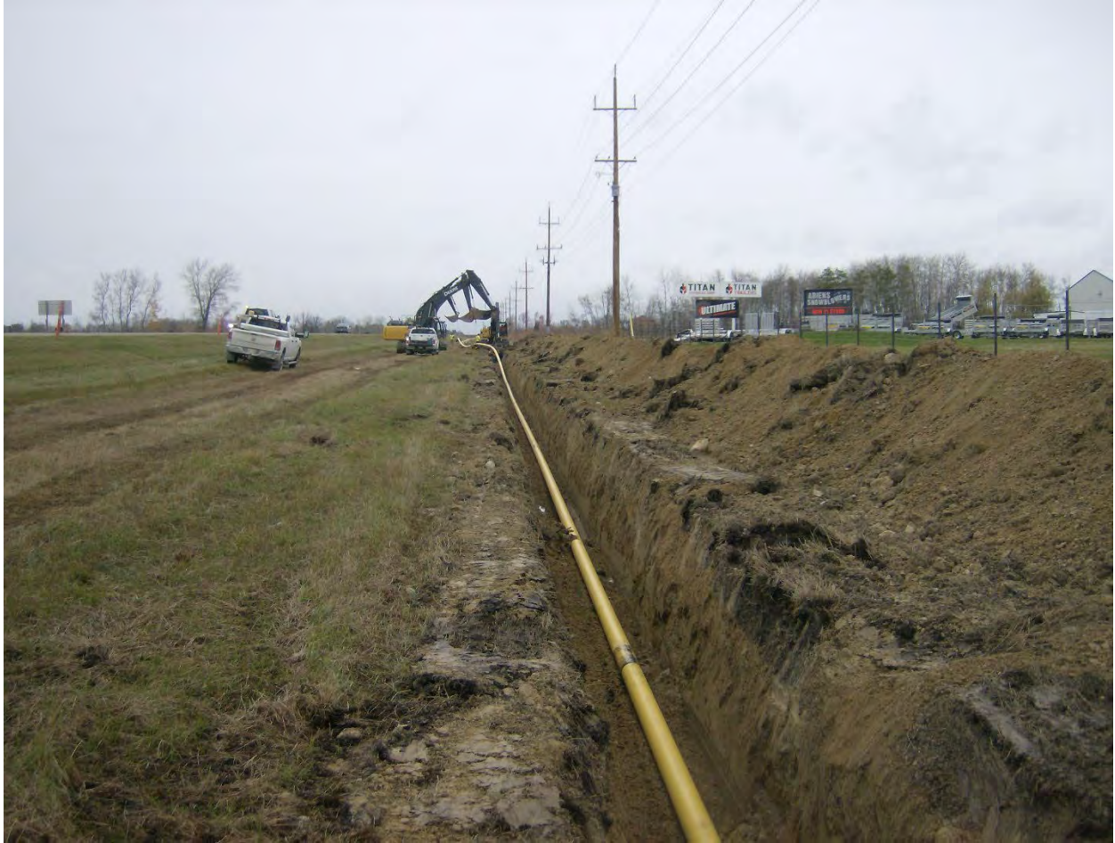
Photo 2-3: Trenching and lowering in pipe
