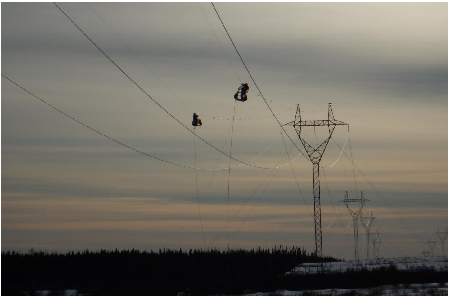
Photo 3: Bird diverter installation on the Keeyask Transmission Project.
