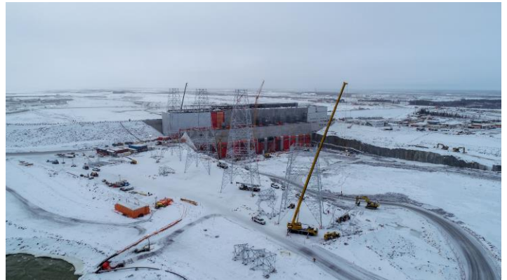
Photo 2: Final tower assembly on the Keeyask Transmission Project.
