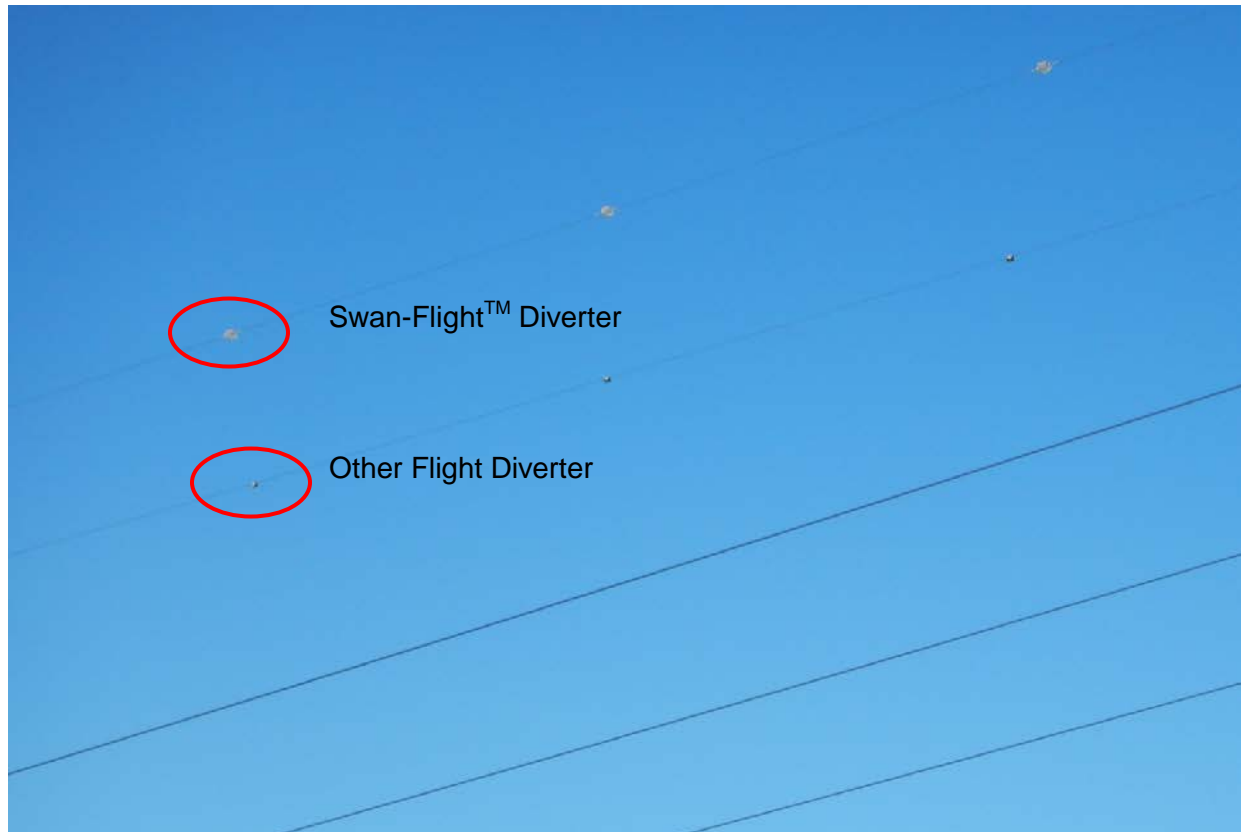
Photo 1. Swan-Flight™ Diverters and other diverters installed on Keeyask Transmission Project's generation outlet transmission line sky wires.
