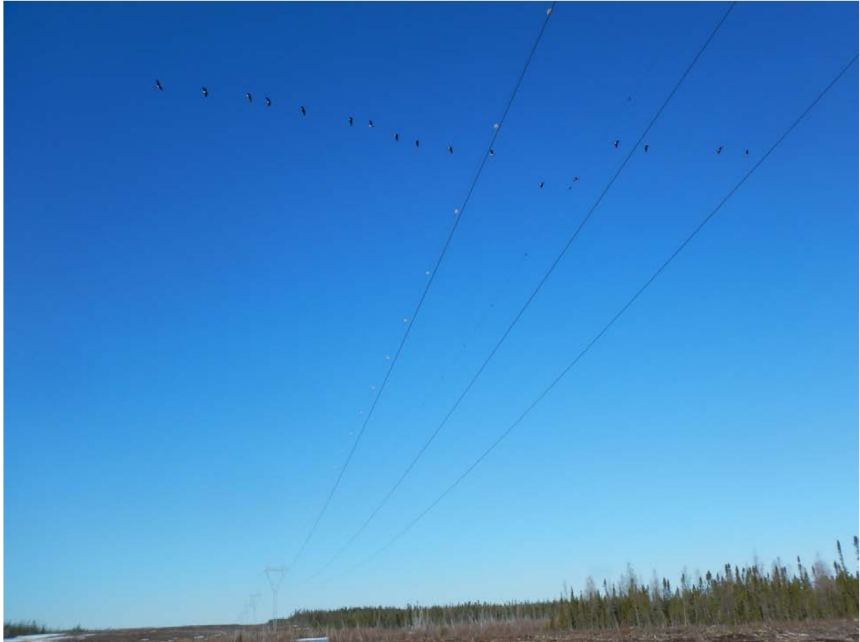
Photo 4. Flock of Canada geese ( Branta canadensis ) flying above the Keeyask Transmission Project's generation outlet transmission lines. Swan Flight™ diverters can be seen on the sky wires.
