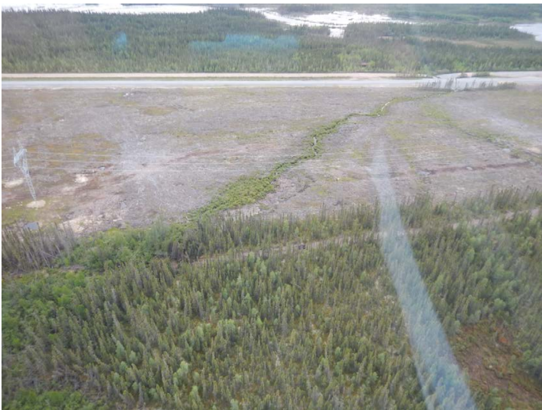
Photo 1. KR1-Aqua-128, KR3-Aqua-129, and KR2-Aqua-130 (tributary of the Butnau River). Un-mitigated stream crossing June 21, 2016 (top) and state as of June 26, 2017 (bottom).
