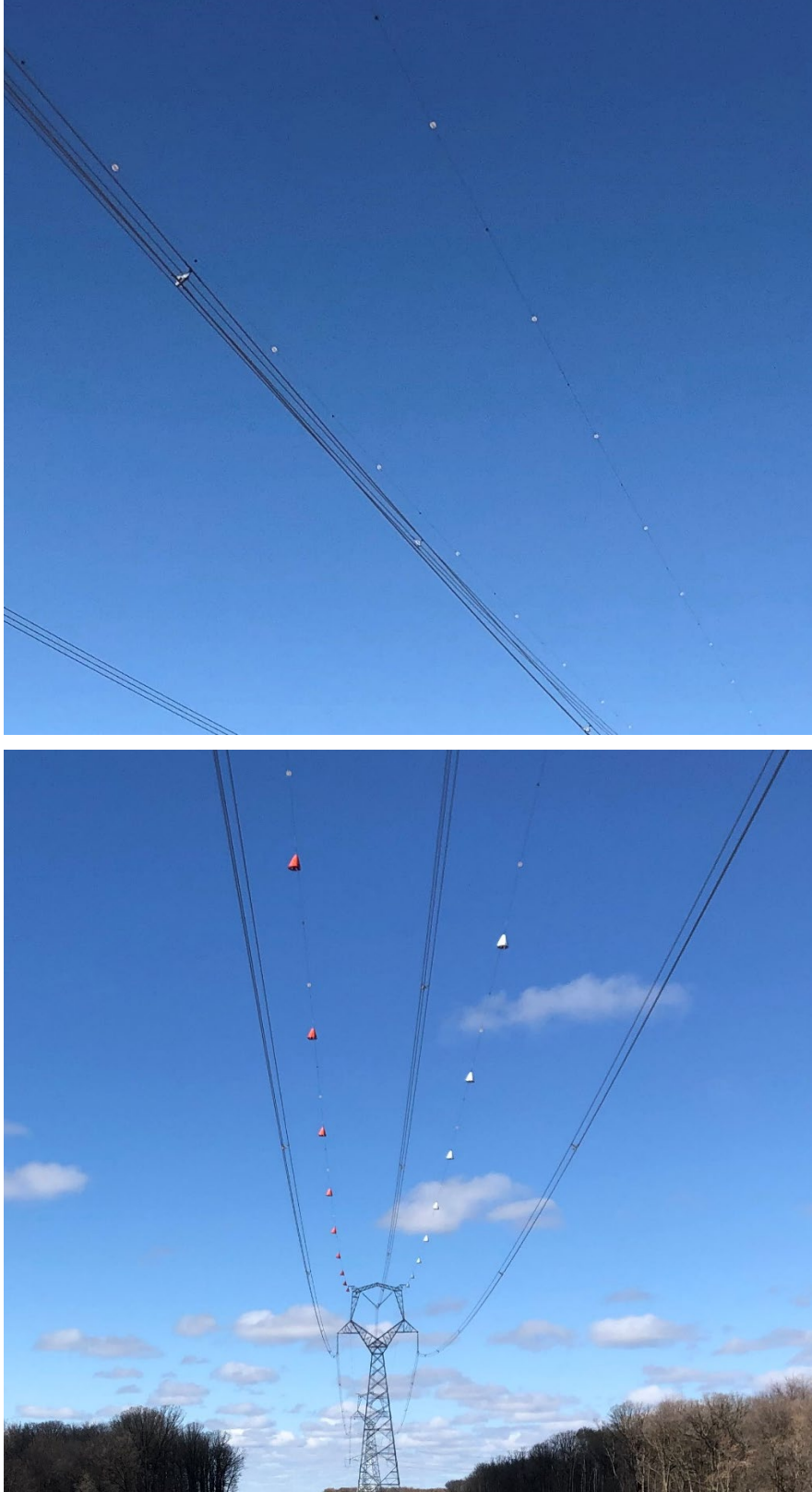
Photo 2. Alternating Swan-Flight Bird Diverters and Bird Flight Bird Diverters (top), and additional aircraft cone markers (bottom) on the Manitoba-Minnesota Transmission Project
