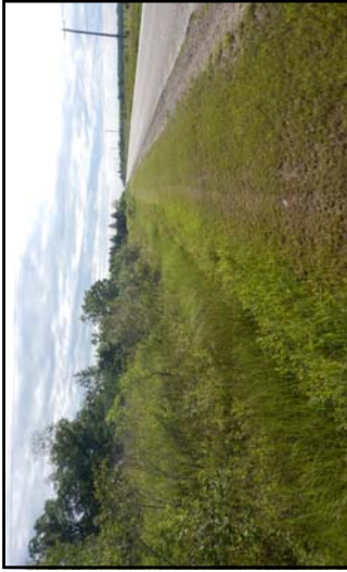
72RT- Facing E, ROW intersection with Dawson rd. Culvert needed to cross steep ditch on both sides of the road to access the ROW. Some clearing req. on both sides of ROW.
