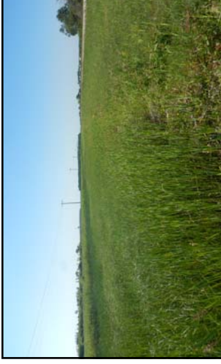
99RT- Facing S. ROW intersection with PTH 89. Culverts needed to cross steep ditch on both sides of road to access ROW.. Clearing req. on E side of ROW.
