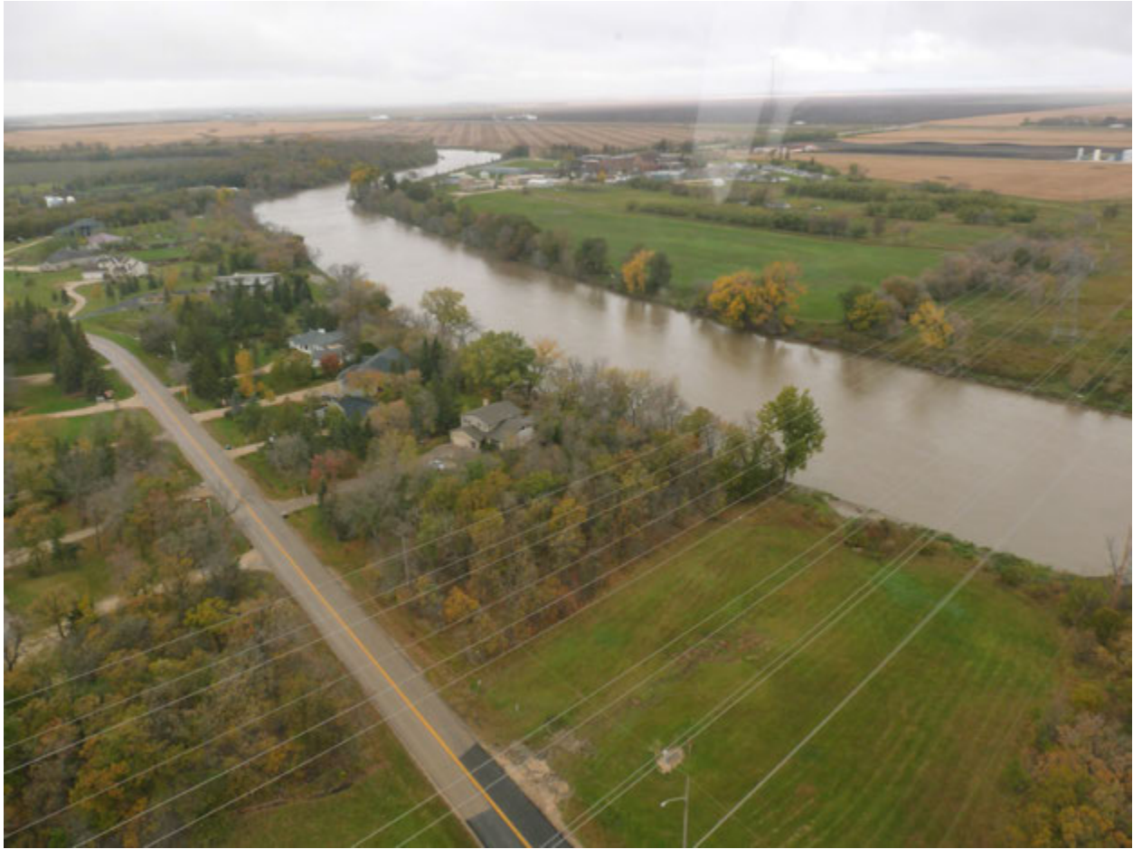
Photo 12. South Loop Transmission Line Corridor and 230 kv line crossing the Assiniboine River.
