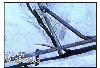
Rebar welded to intersecting rebar to ensure equipotential plane is continuously conductive
