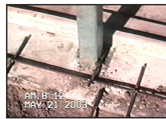
Stanchion bonded by welding a piece of rebar to its base and to the rebar that forms the equipotential plane.
