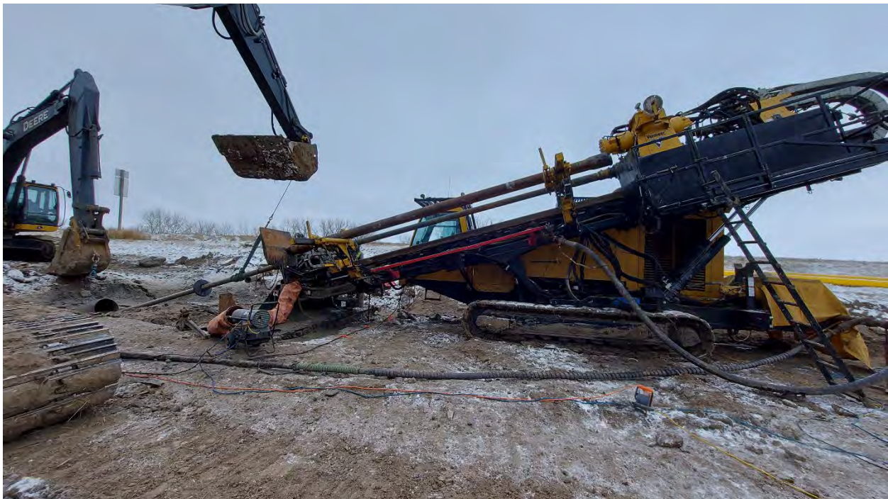
Photo 2-5: Horizontal directional drill of entry/exit hole.
