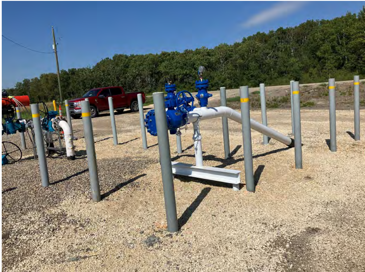
Figure 9-4 Typical above-ground control point showing limited area of gravel pad around the exposed facility
