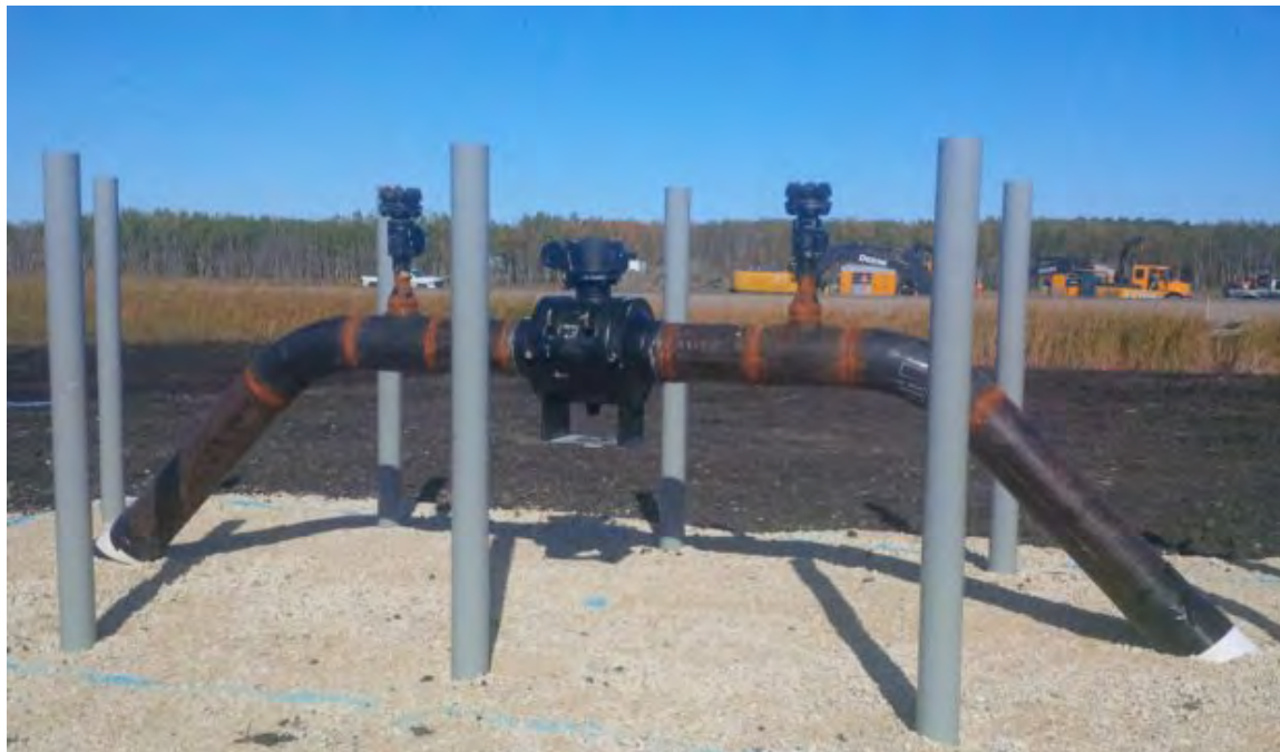
Photo 2-4: Example of control point with valves prior to paint application. In this example no tie-in is shown, only a control point on a single gas pipeline.
