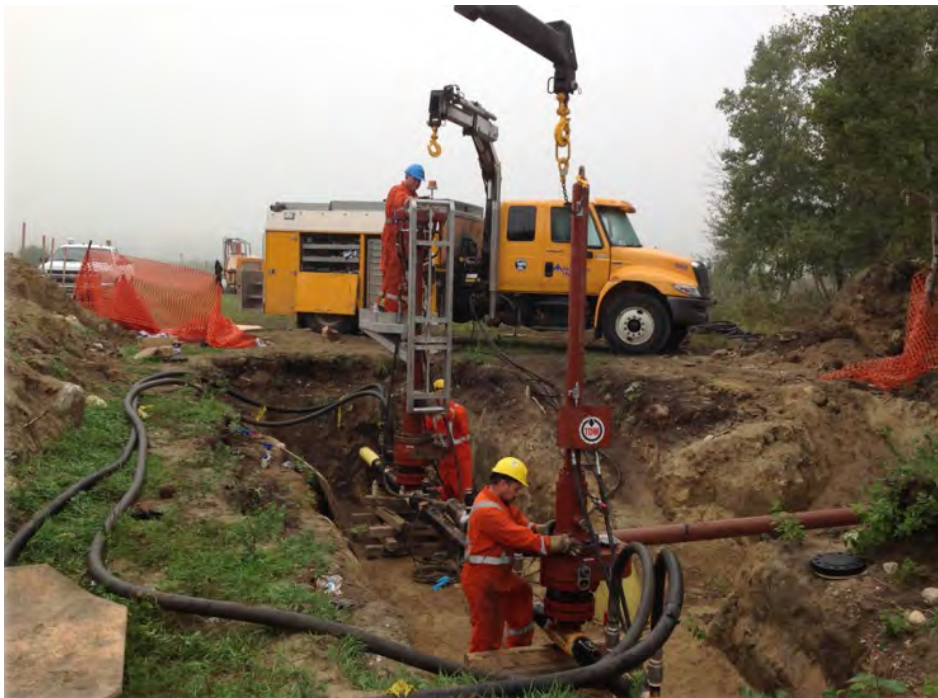
Photo 2-7: Example of hot tap fitting installation and bypass hoses
