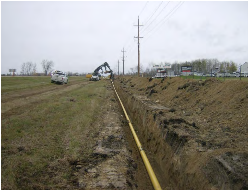
Photo 2-6: Example of an excavated trench and lowering in steel pipe
