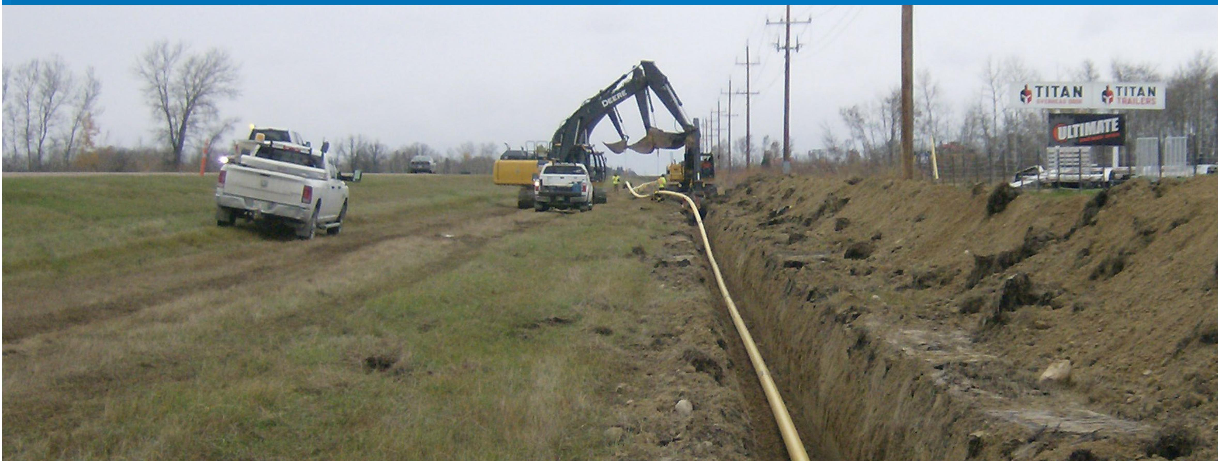
**Trenching** involves digging a long narrow hole in the ground and placing the pipeline within it.
