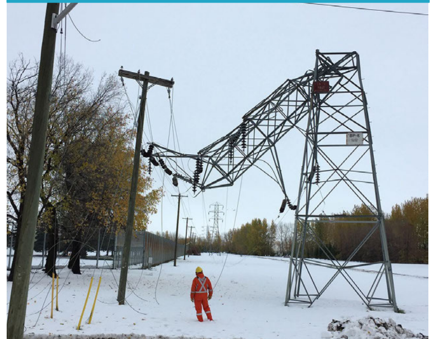
Damaged tower in Portage la Prairie
