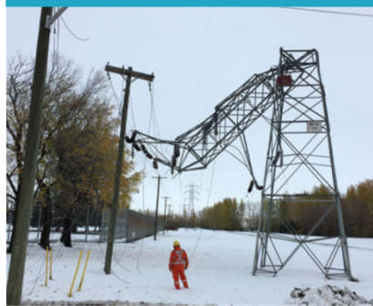
Damaged tower in Portage la Prairie
