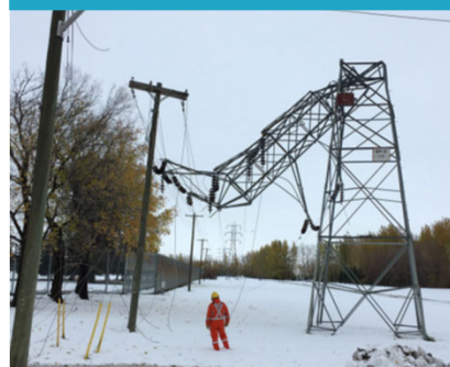
Damaged tower in Portage la Prairie
