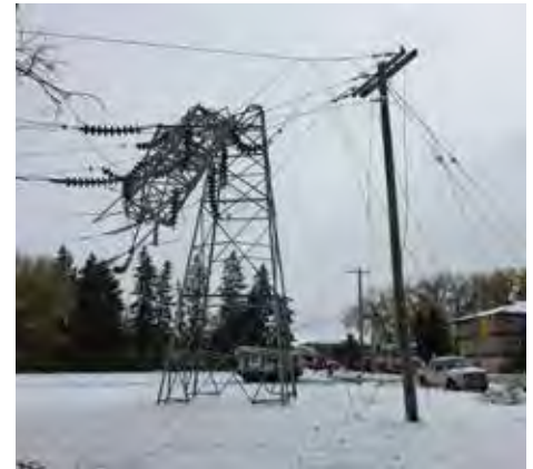
A steel tower in the Portage la Prairie area left crumpled by the storm.
