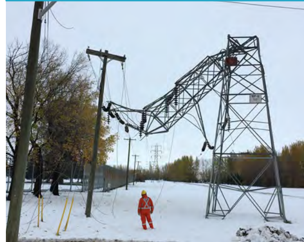
Damaged tower in Portage la Prairie
