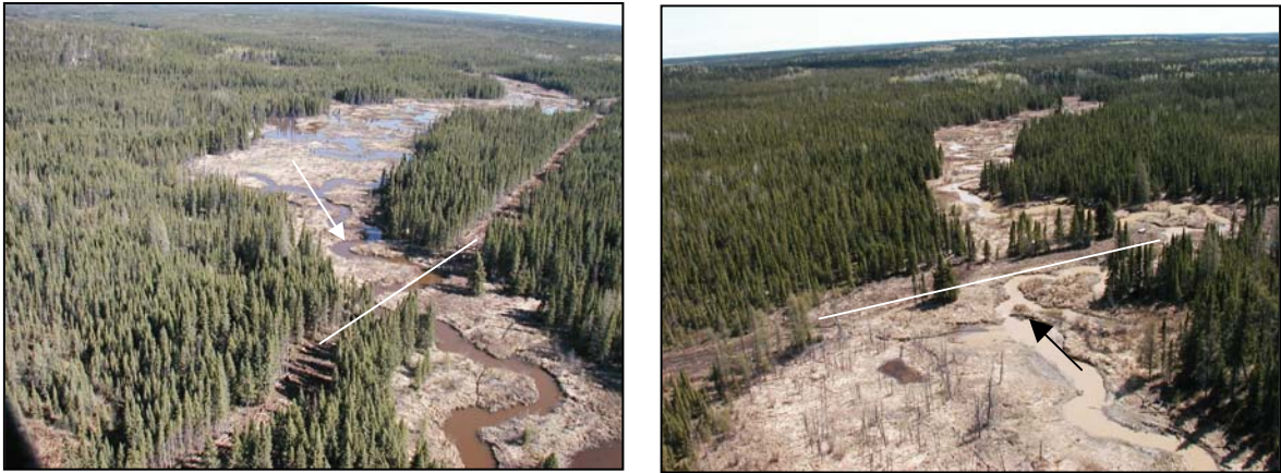
Figure 6.6-13. Aerial view of road crossing at R5 (left) and at R8 (right). Line indicates crossing location; arrow indicates direction of water flow.
