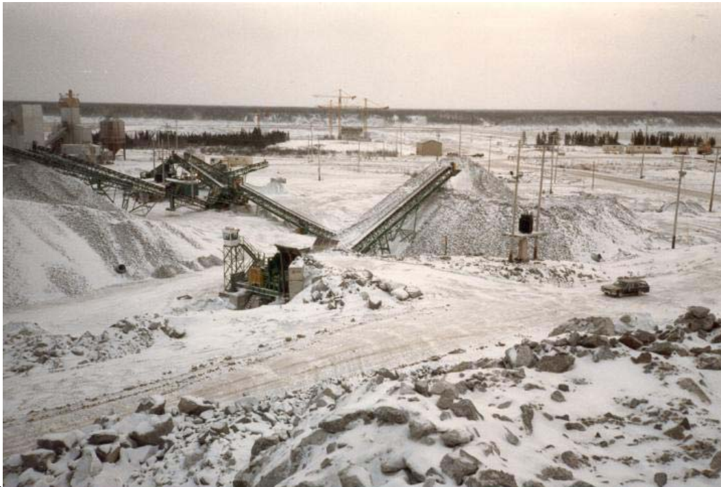
Figure 4.6-12 Typical Rock Crusher Operation
