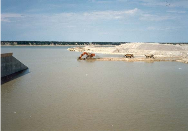
Figure 4.6-19 Typical cofferdam removal with backhoe
