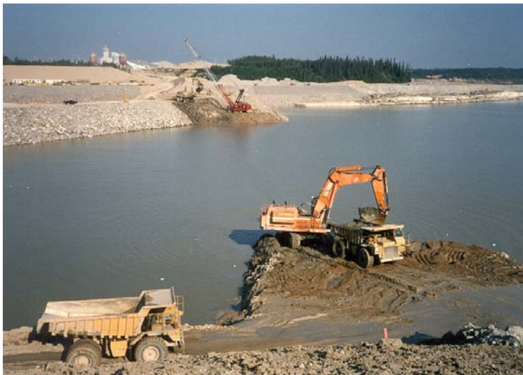
Figure 4.6-18 Typical cofferdam removal with backhoe
