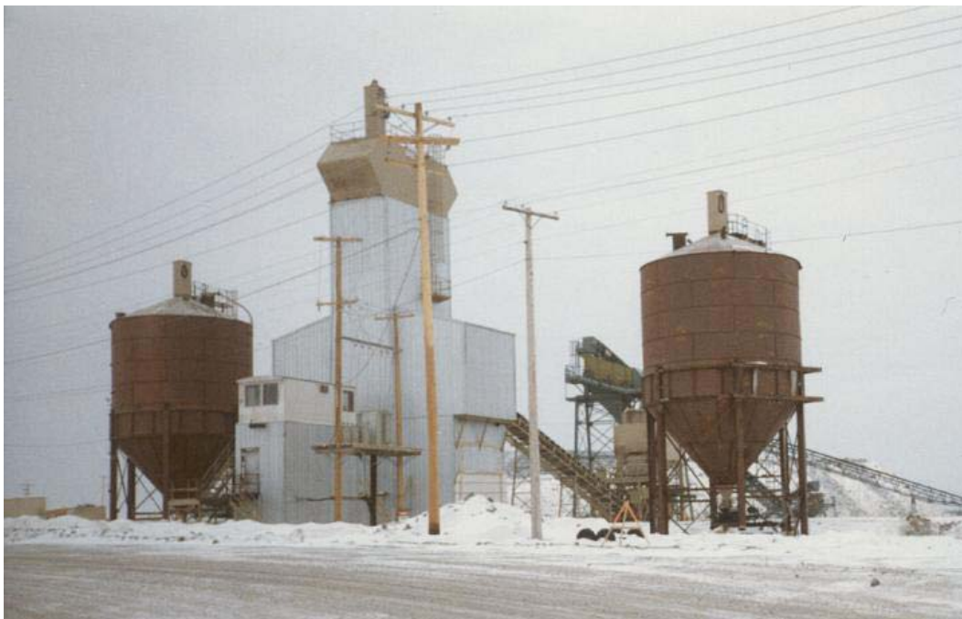
Figure 4.6-11 Typical Concrete Batch Plant and Cement Storage Silos
