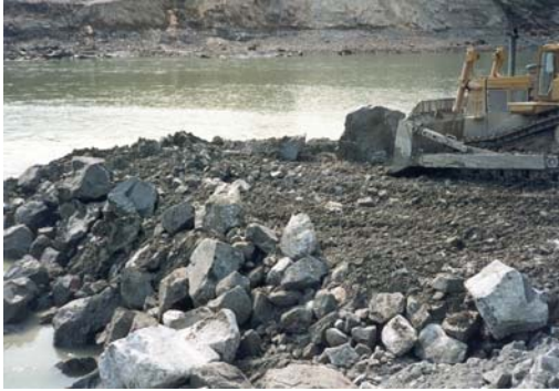
Figure 4.6-14 Typical cofferdam being pushed into the river channel.
