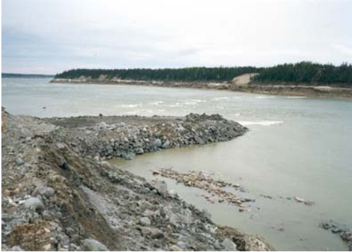
Figure 4.6-15 Typical cofferdam advanced into the river channel
