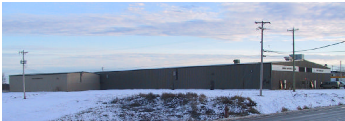
Figure 2.49 The Gilbert McDonald Arena in Nelson House
