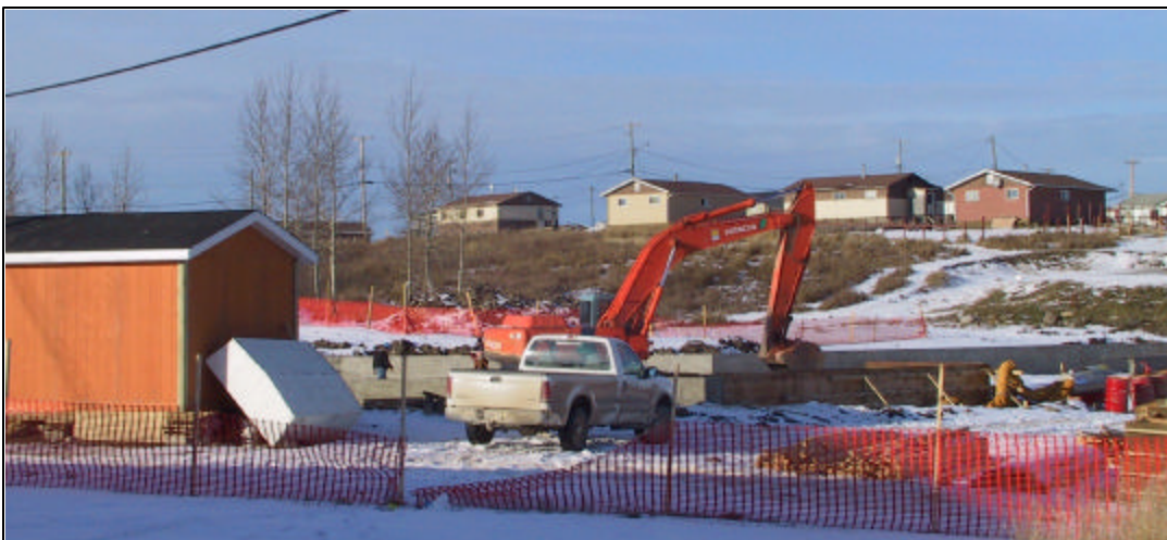
Figure 2.45 Construction of the Elders Care Home in Nelson House
