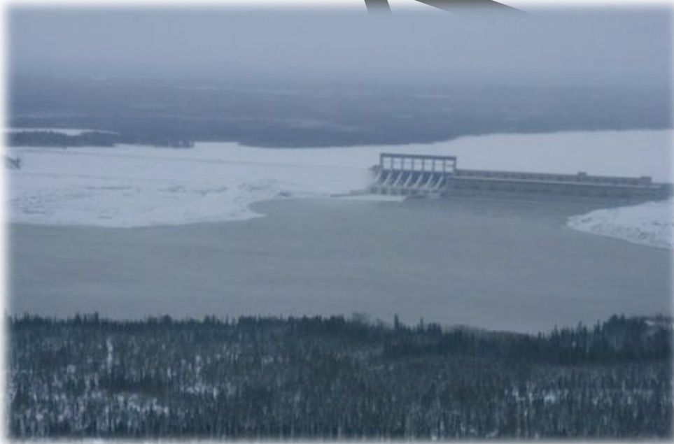
Figure 4 – Aerial view of Limestone Generating Station. Photo Credit: Brian Kotak
