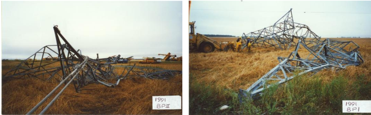
Photo 2.2-1: Damaged Towers of (TWG #1991) Bipole I and II Lines by Downburst Winds in 1996
