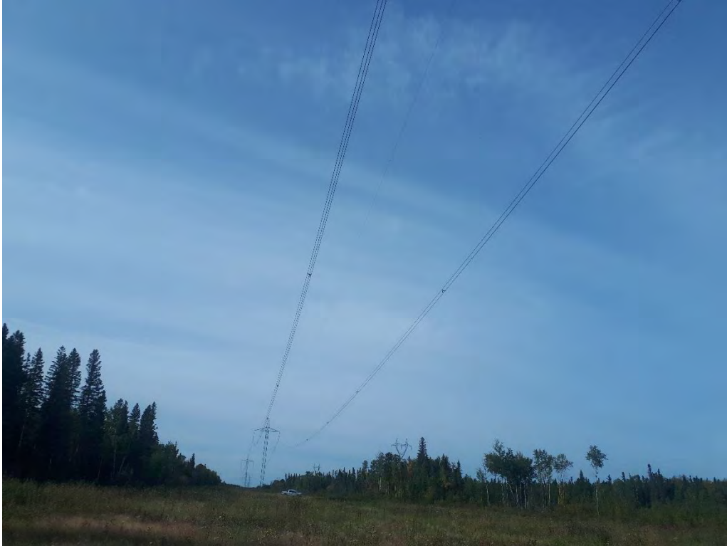
Transmission line without bird diverters installed
