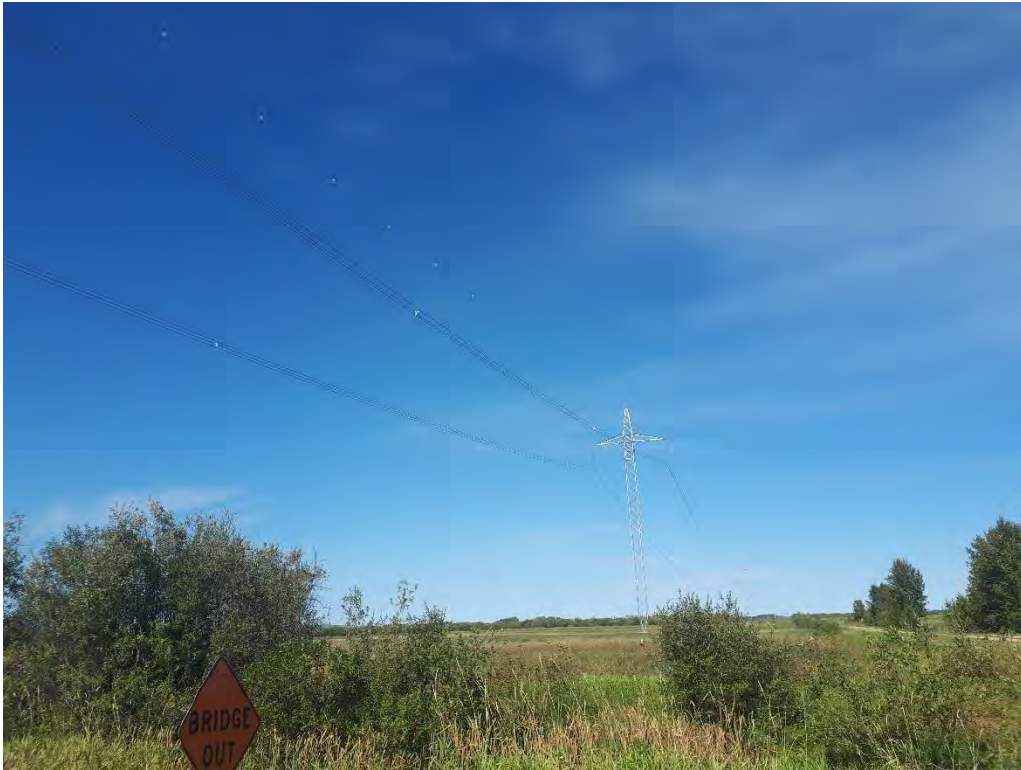
Transmission line with bird diverters installed
