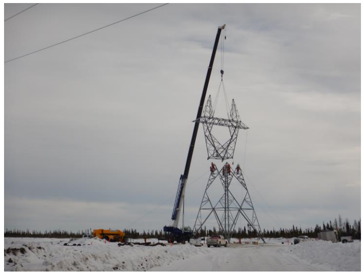
Photo 3: Tower assembly on the Keeyask Transmission Project.
