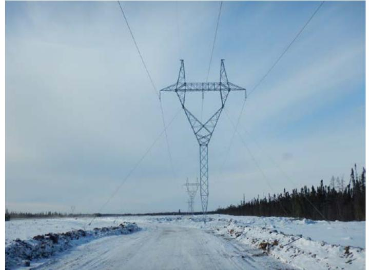
**Photo 7: Completed Keeyask Transmission Tower Assembly and Stringing**
