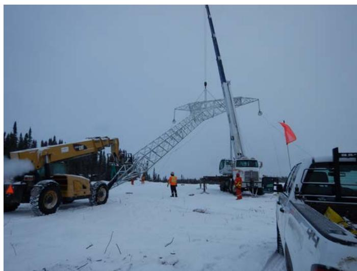
**Photo 3: Keyask Transmission Tower Erection**
