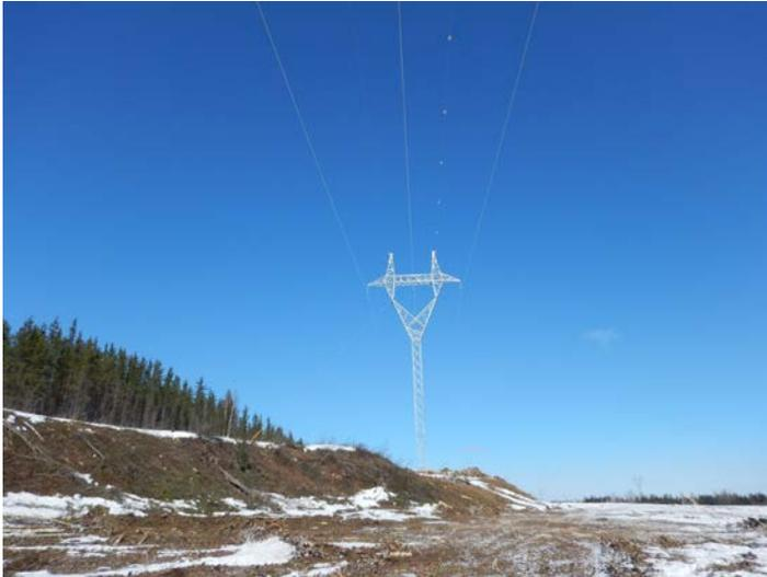
**Photo 6: Keeyask Transmission Line with Bird Diverters**
