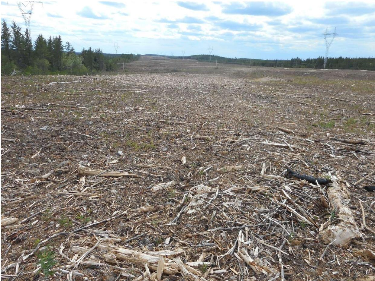
**Photo 3-1: Example of minimal exposure of mineral substrates in cleared ROW**
