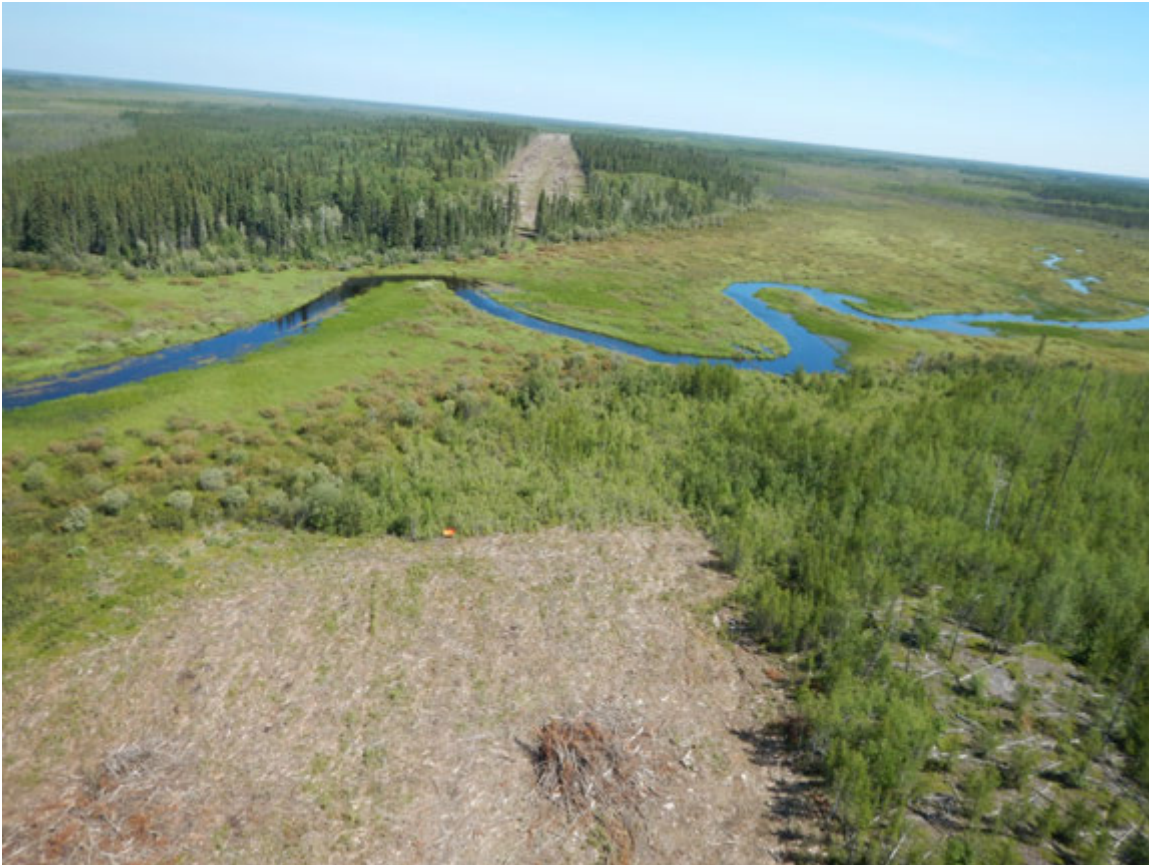
Photo 8-3 Newly cleared ROW at watercourse crossing showing riparian buffer
