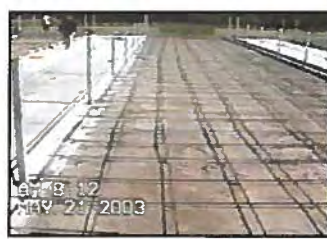
Equipotential planes using rebar in the milking parlour and loafing area, in position before concrete is placed. A grid size of 15 cm x 15 cm (6 in. x 6 in.) is recommended for the milking parlour, 30 cm x 30 cm (12 in. x 12 in.) elsewhere.
