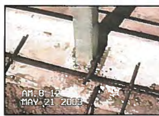
Stanchion bonded by welding a piece of rebar to its base and to the rebar that forms the equipotential plane.
