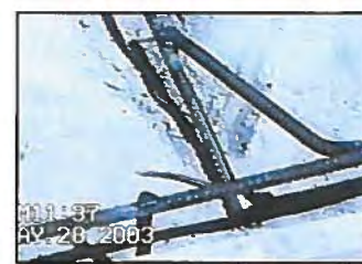
Rebar welded to intersecting rebar to ensure equipotential plane is continuously conductive
