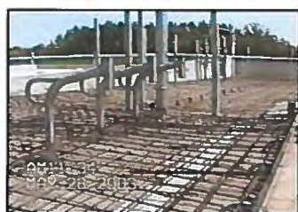
Equipotential planes using rebar in the milking parlour and loafing area, in position before concrete is placed. A grid size of 15 cm x 15 cm (6 in. x 6 in.) is recommended for the milking parlour, 30 cm x 30 cm (12 in. x 12 in.) elsewhere.
