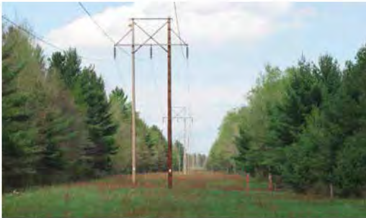
Figure 3. Examples of high quality (top) and poor quality (bottom) golden-winged warbler habitat in a transmission line ROW ((GWWAWG (2013). Photos credits from top and bottom: Sara Barker Swarthout; and Amber Roth)
