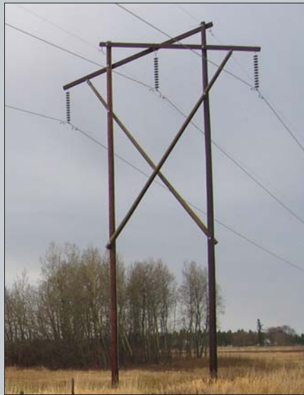
A single circuit transmission line consists of a set of three conductors to create a complete electrical circuit
