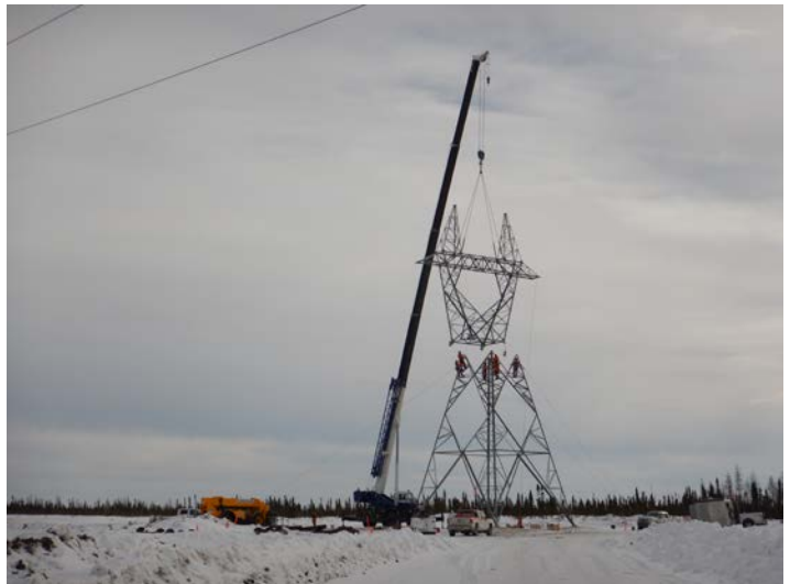
Photo 3: Tower assembly on the Keeyask Transmission Project.
