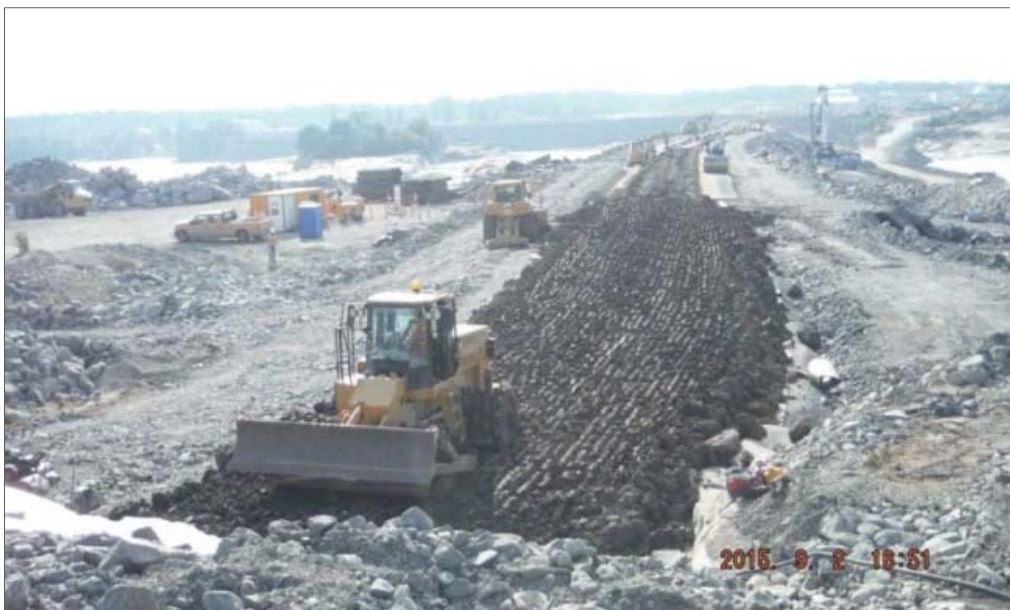
Photo 2: Class 1, 3 and 4 material being placed on Main Dam (September 2, 2015)
