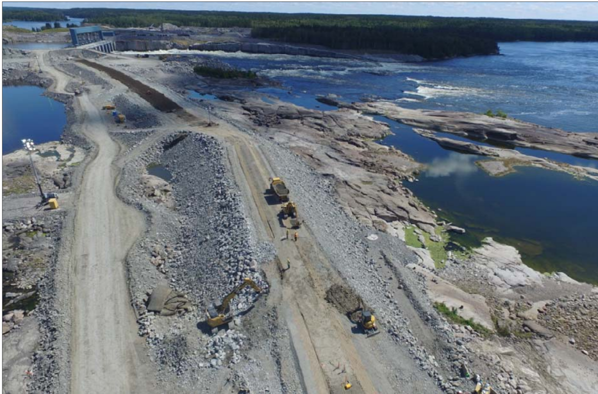
Photo 2: Class 1, 3 and 4 material being placed on Main Dam (September 2, 2015)
