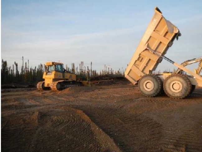
Photo 5: Keewatinohk Converter Station - Leveling backfill material
