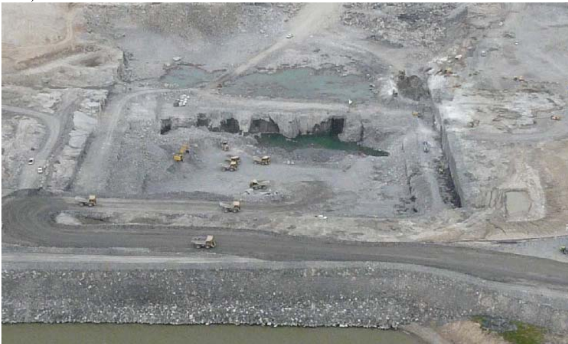
Photo 3: Rock Excavation inside the Powerhouse Cofferdam looking upstream (September 2015)
