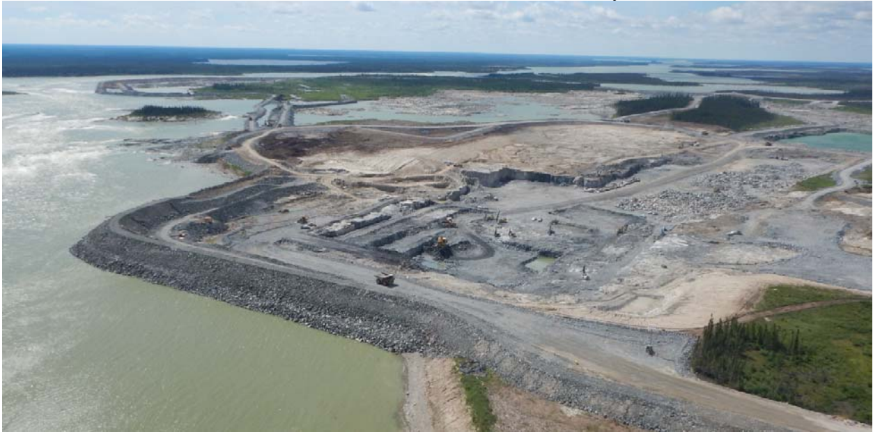
Photo 2: Rock Excavation inside the Powerhouse Cofferdam (July 27, 2015)
