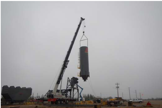
Photo 6: Keewatinohk Converter Station – Installation of concrete batch plant
