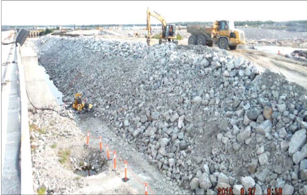
Photo 3: South Dam under Construction (August 27, 2015)
