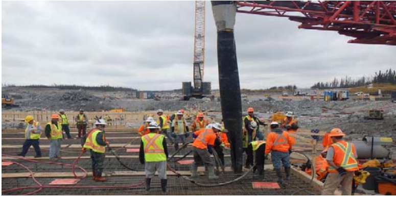
Photo 4: First Concrete Placement (September 26, 2015)
