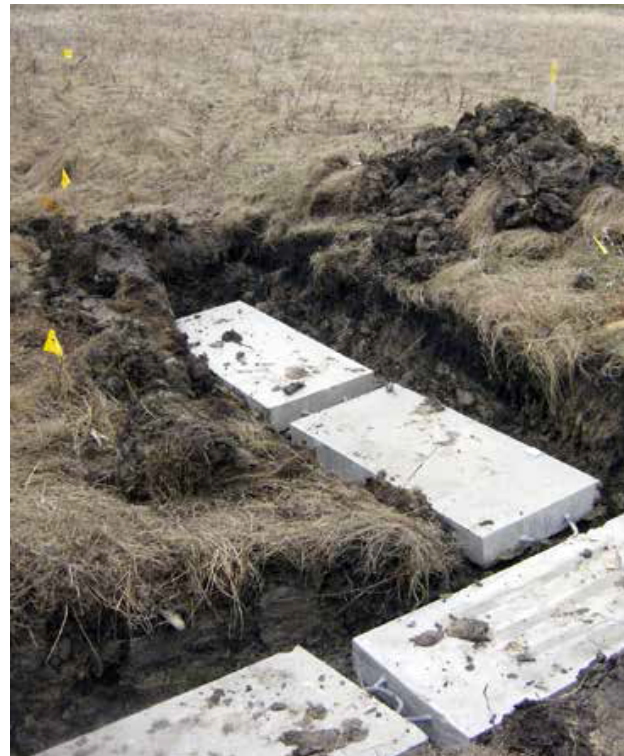
FIGURE 12 – INSUFFICIENT COVER REMEDIATION: INSTALLATION OF REPLACEMENT LINE (LEFT) AND INSTALLATION OF CONCRETE SLABS OVER PIPELINE (RIGHT)
