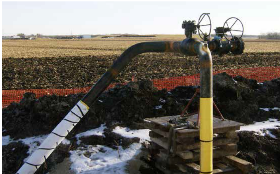
FIGURE 35 – PIG LAUNCHER INSTALLATION
