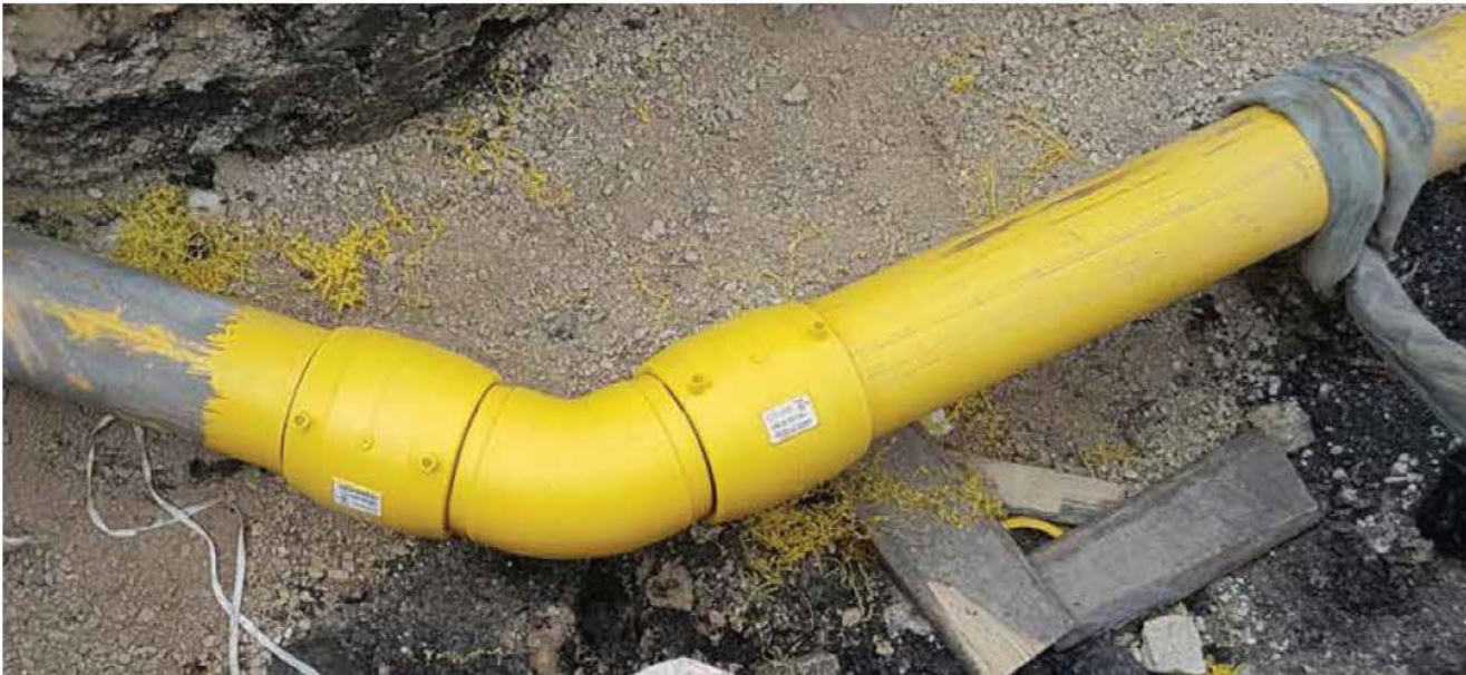
FIGURE 31 – WAVERLEY WEST PHASE 1 UTILIZED NPS 8 POLYETHYLENE PIPE
