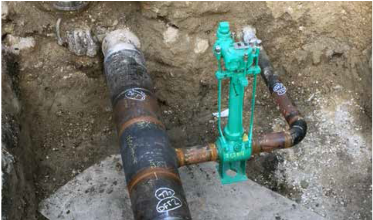
FIGURE 11 – REPLACEMENT STATION ISOLATION VALVE
