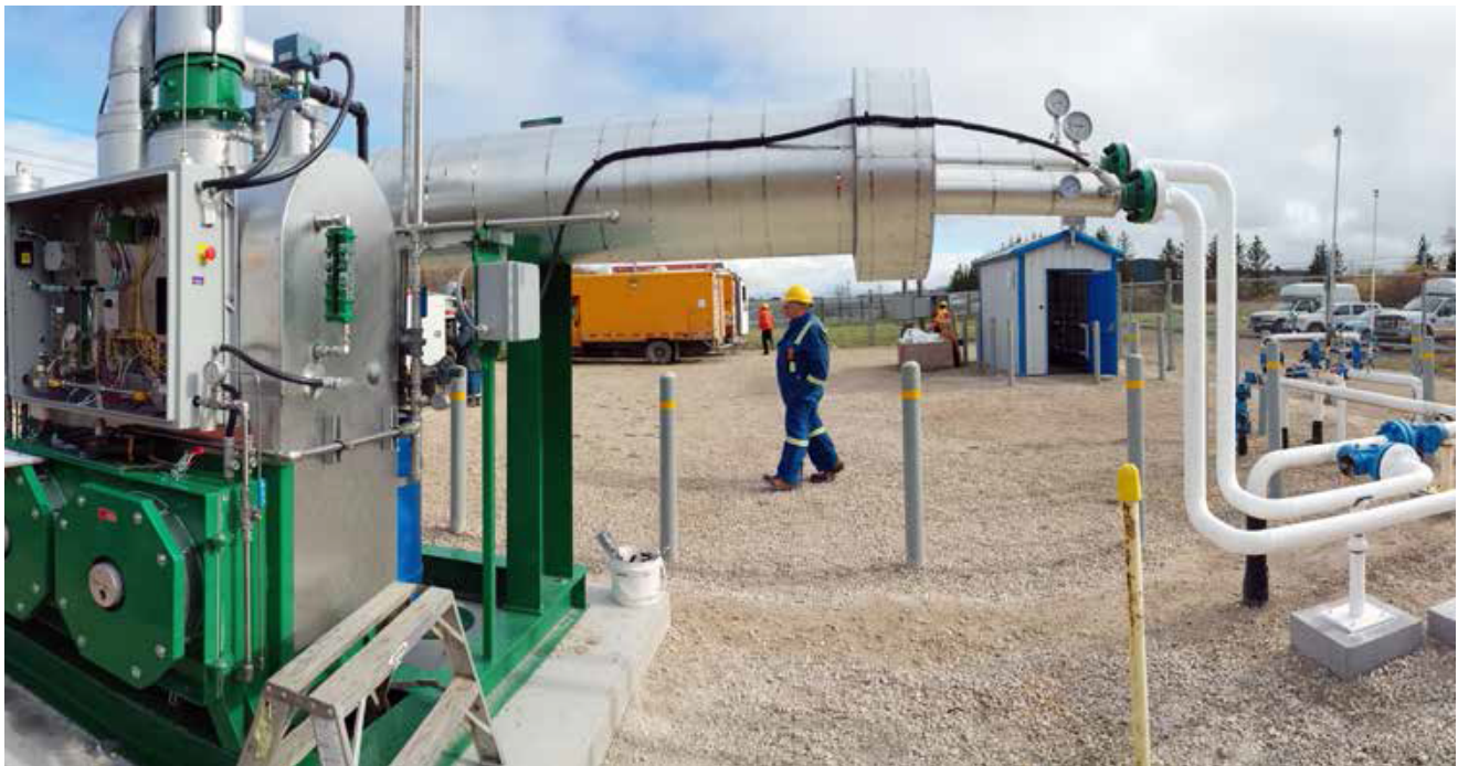
FIGURE 22 – LINE HEATER
