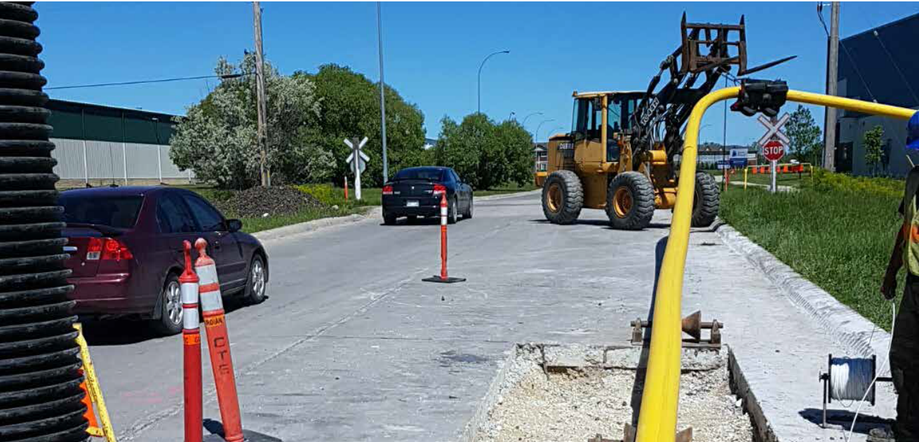
FIGURE 4 – 219.1MM (8") POLYETHYLENE (PE) FOR A NEW CUSTOMER
