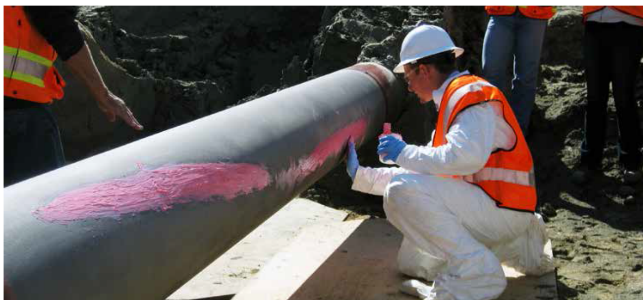
FIGURE 8 – PIPE DEFECT REPAIR
