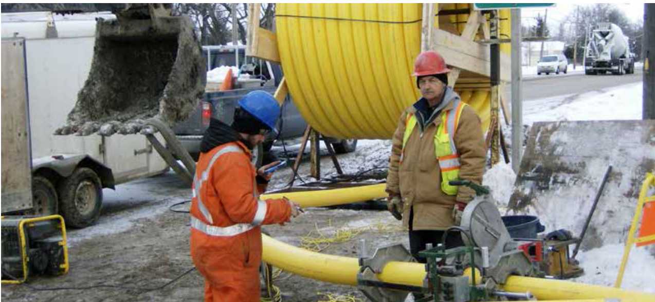
FIGURE 16 – INSTALLATION OF NPS 6 PE MAIN UNDER BUNNS CREEK AT HENDERSON HIGHWAY, WINNIPEG
