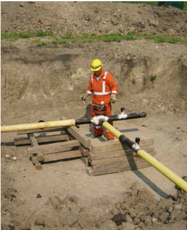
FIGURE 12 – INSUFFICIENT COVER REMEDIATION: INSTALLATION OF REPLACEMENT LINE (LEFT) AND INSTALLATION OF CONCRETE SLABS OVER PIPELINE (RIGHT)
