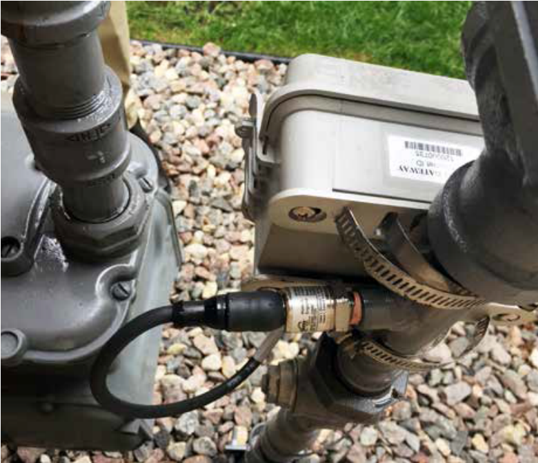
FIGURE 39 – REMOTE SENSING UNIT
