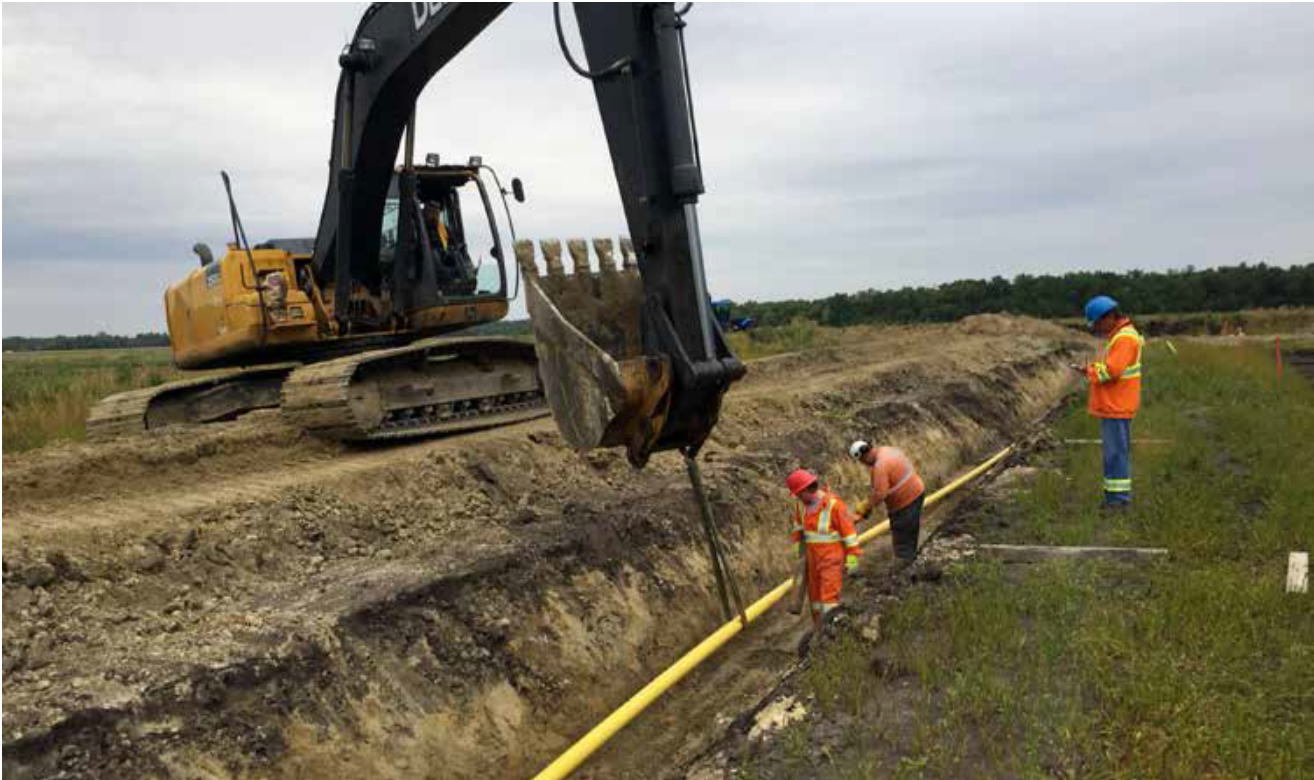
FIGURE 42 – ST. PIERRE 114.3MM (4") TRANSMISSION PRESSURE UPGRADE
