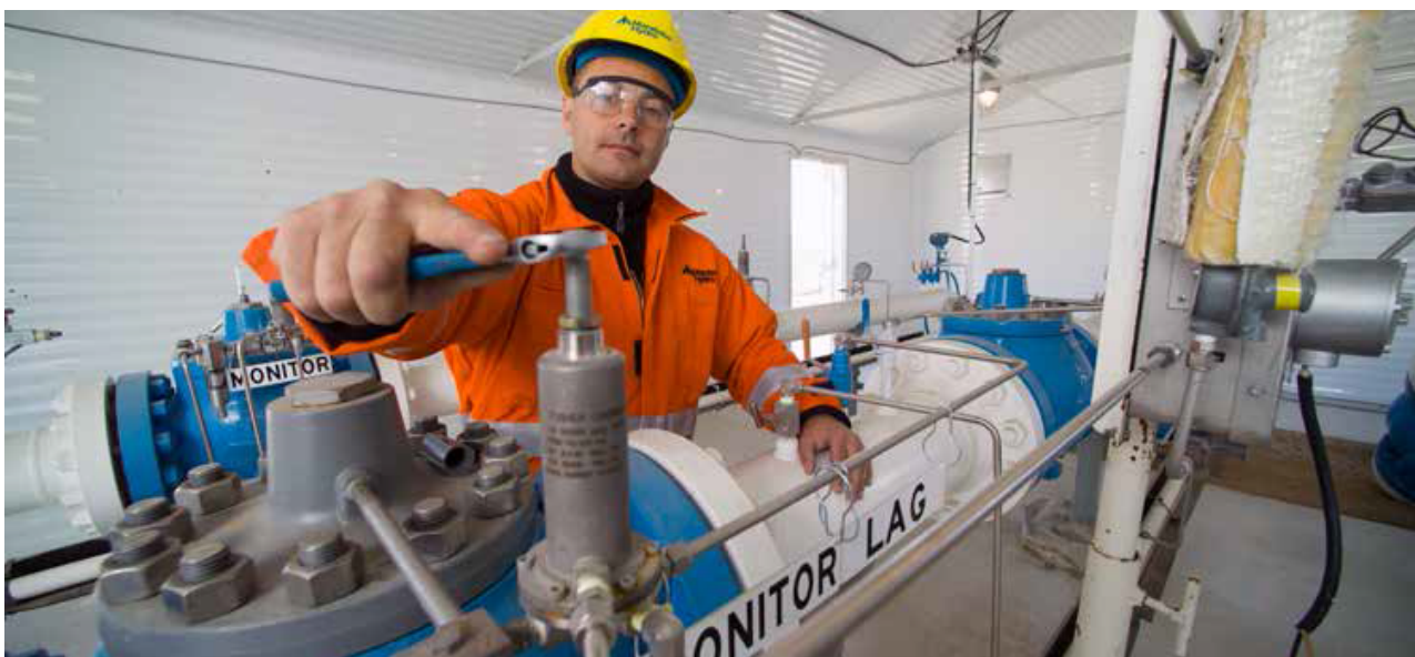
FIGURE 27 – MAINTENANCE OF GAS PRESSURE REGULATION EQUIPMENT IN A REGULATING STATION
