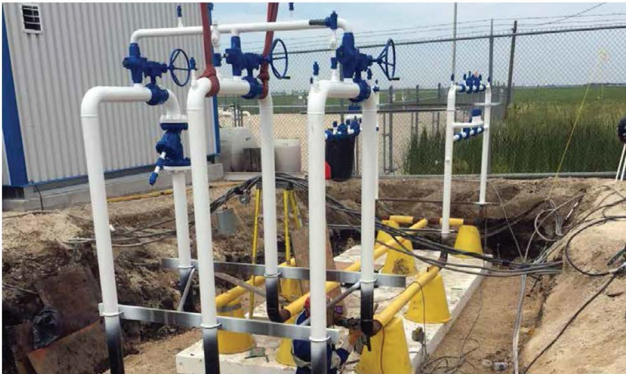
FIGURE 1 – CONSTRUCTION OF A NEW PRESSURE REGULATING STATION
