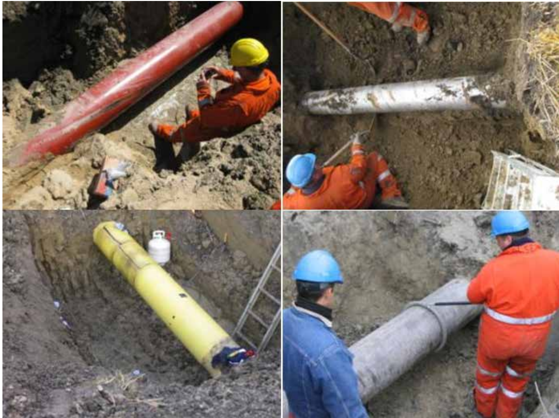
Figure 2: Various types of coatings on steel pipelines: fusion bonded epoxy (top left), paraffin wax (top right), polyethylene, informally yellow jacket (bottom left) and coal tar enamel (bottom right).
