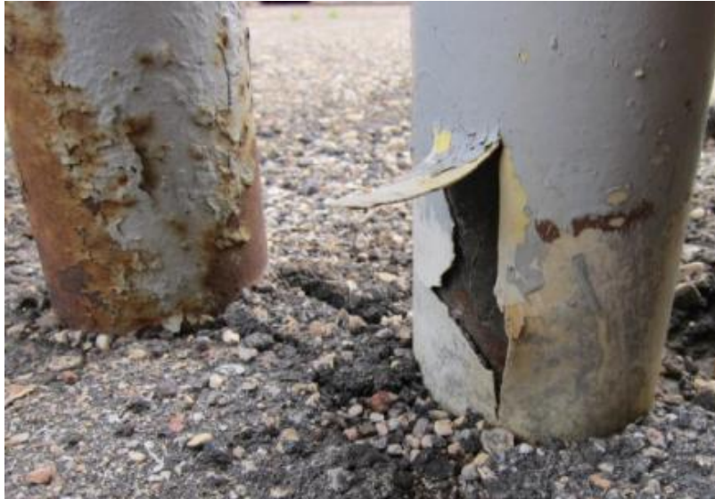
Figure 3: Blistering and cracked coating of risers without sleeving
