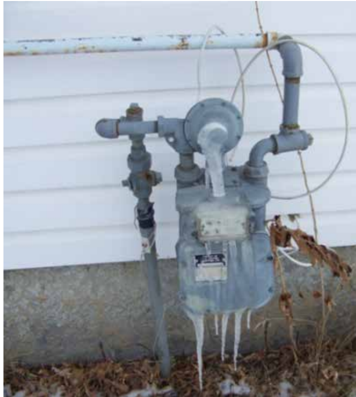
Figure 14: Frozen over relief vent on residential meter set
