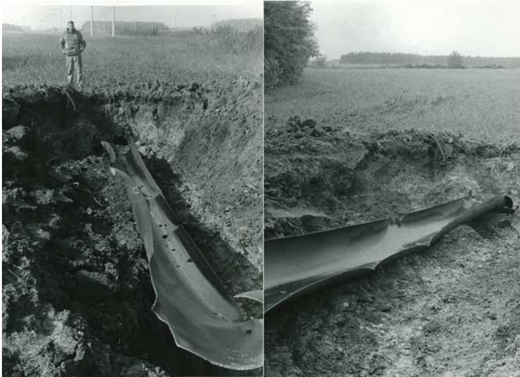
Figure 12: Rupture incident of La Salle NPS 12 transmission pipeline south of McGillivray Boulevard during pneumatic pressure test in 1964. Rupture occurred at 7080 kPa (1027 psi) corresponding to 57% SMYS.
